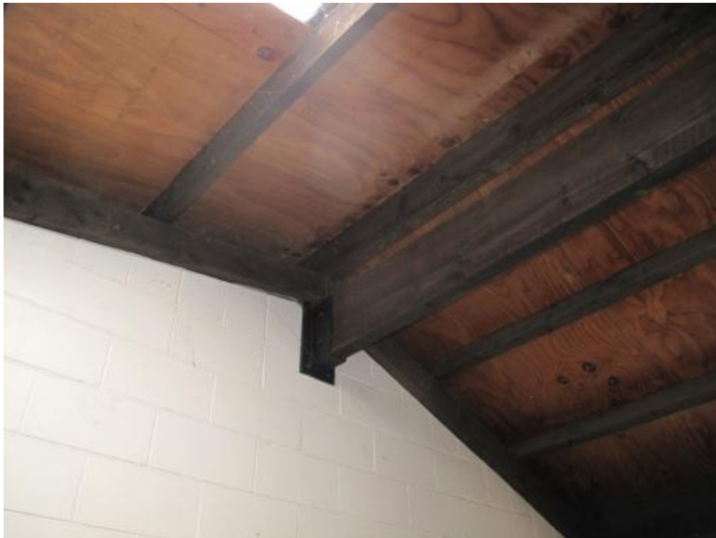
Photograph 12 Bolted brackets supporting timber ridge beam.
