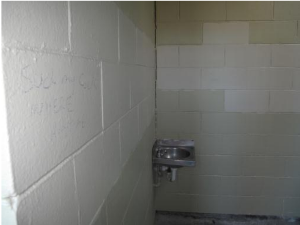
Photograph 5 Gap between Wall 10 and Wall 5, from the south side.
