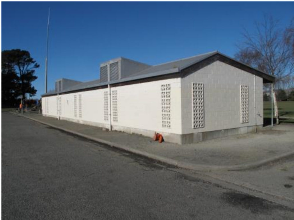
Photograph 2 View of the toilet block from the northwest.
