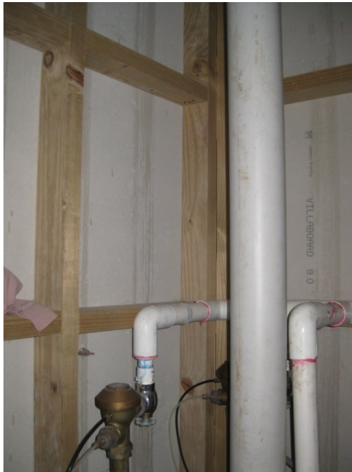
Photo 13: interior view of the services room showing the timber framing and the Villaboard interior lining.
