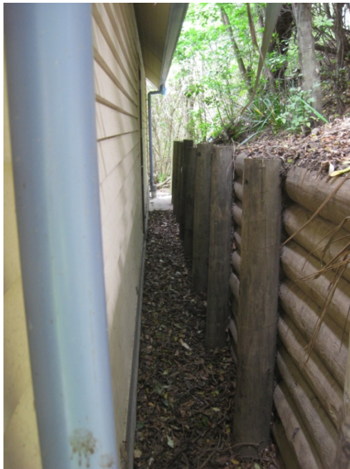
Photo 3: View along the Northwest elevation showing the timber retaining post retaining wall
