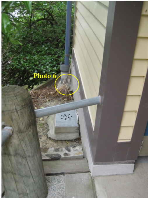
Photo 5: View of the south corner of the building showing cracks between the drains and the building
