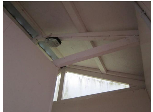
Photo 12: Timber roof trusses at 850mm centres
