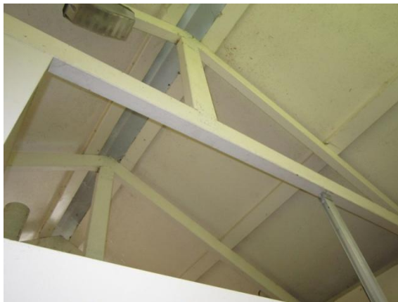
Photo 11: Timber roof trusses at 850mm centres
