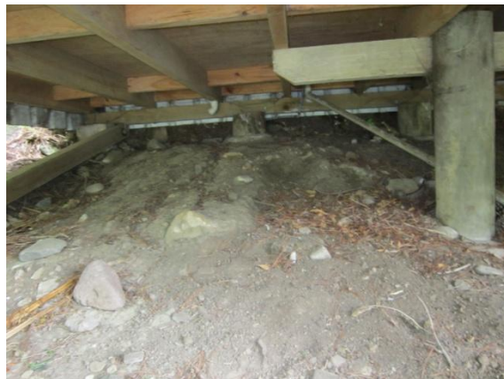
Photo 7: Timber joists, piles and diagonal bracing shown at foundation level (sloping ground)
