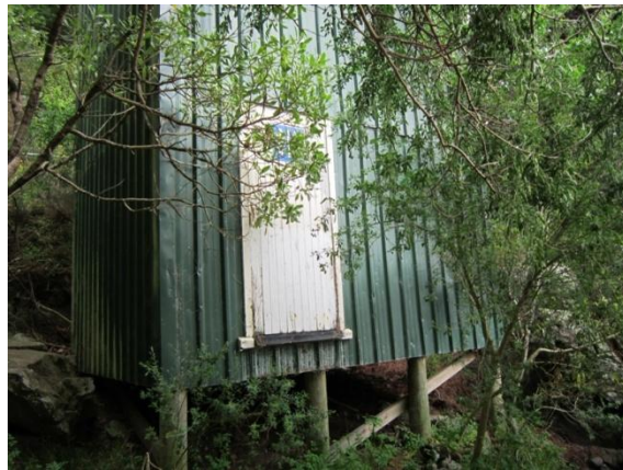
Photo 5: Entrance to ground floor (inaccessible), also showing diagonal timber brace at foundation level
