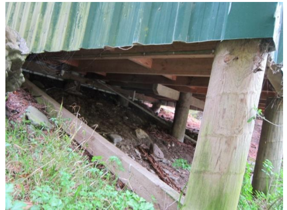
Photo 6: Timber joists, piles and diagonal bracing shown at foundation level (sloping ground)
