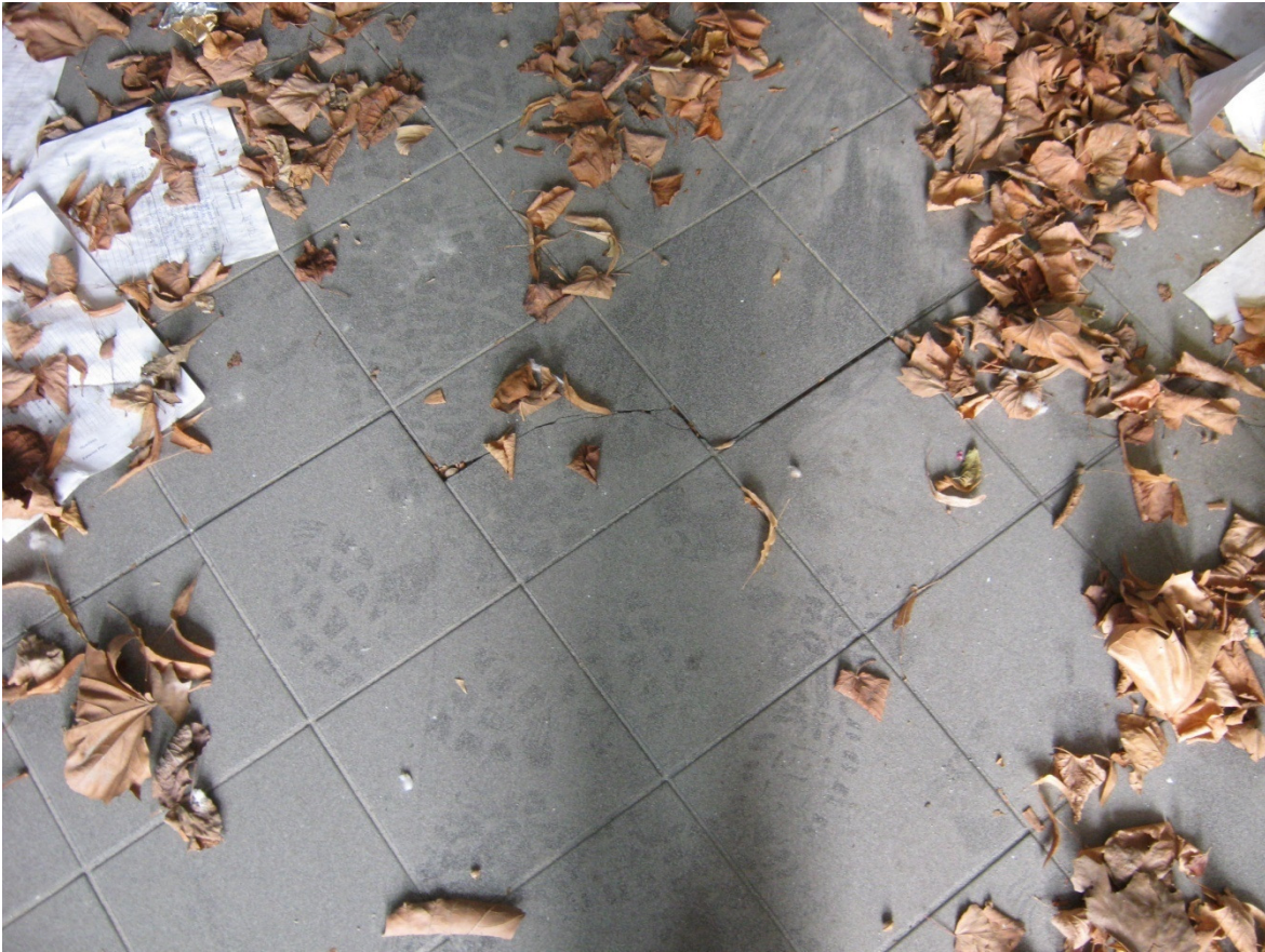
Photograph 3. Small crack in floor tile inside Women's Toilets (Ground Level).
