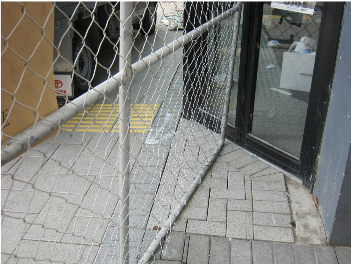
Photograph 4. Some movement in the pavers outside the toilet building entrance.
