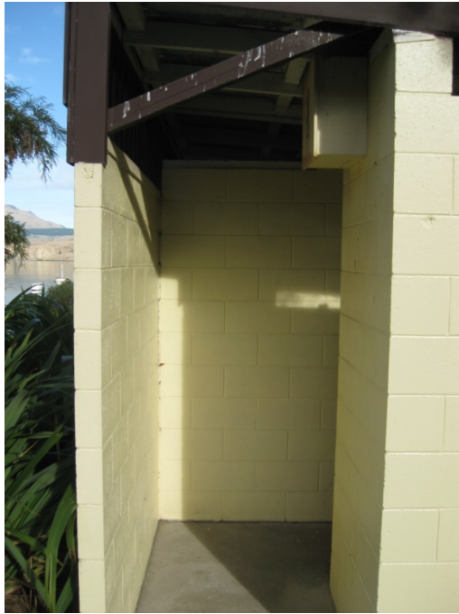
Photo 5: Typical Entrance Detail
