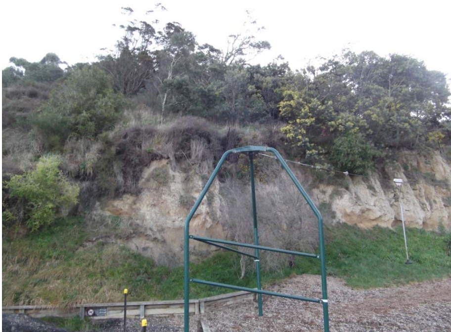
■ Figure 8 Loess cut faces behind the building standing near vertical and stable
