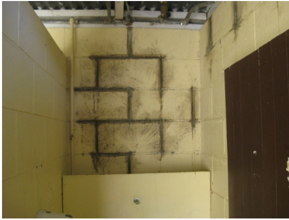
Photo 13: West Wall in Ladies – Mortar Joints appear to have been Re-pointed
