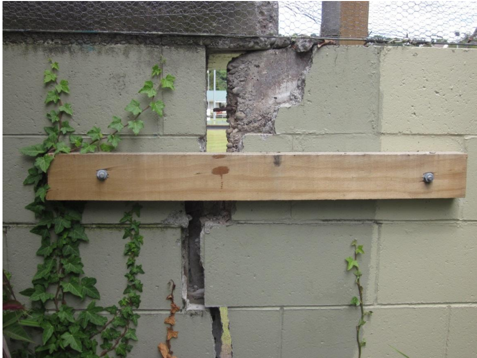
Photograph 7: Cracking to the masonry boundary wall found during the initial inspection on 15 February 2012.
