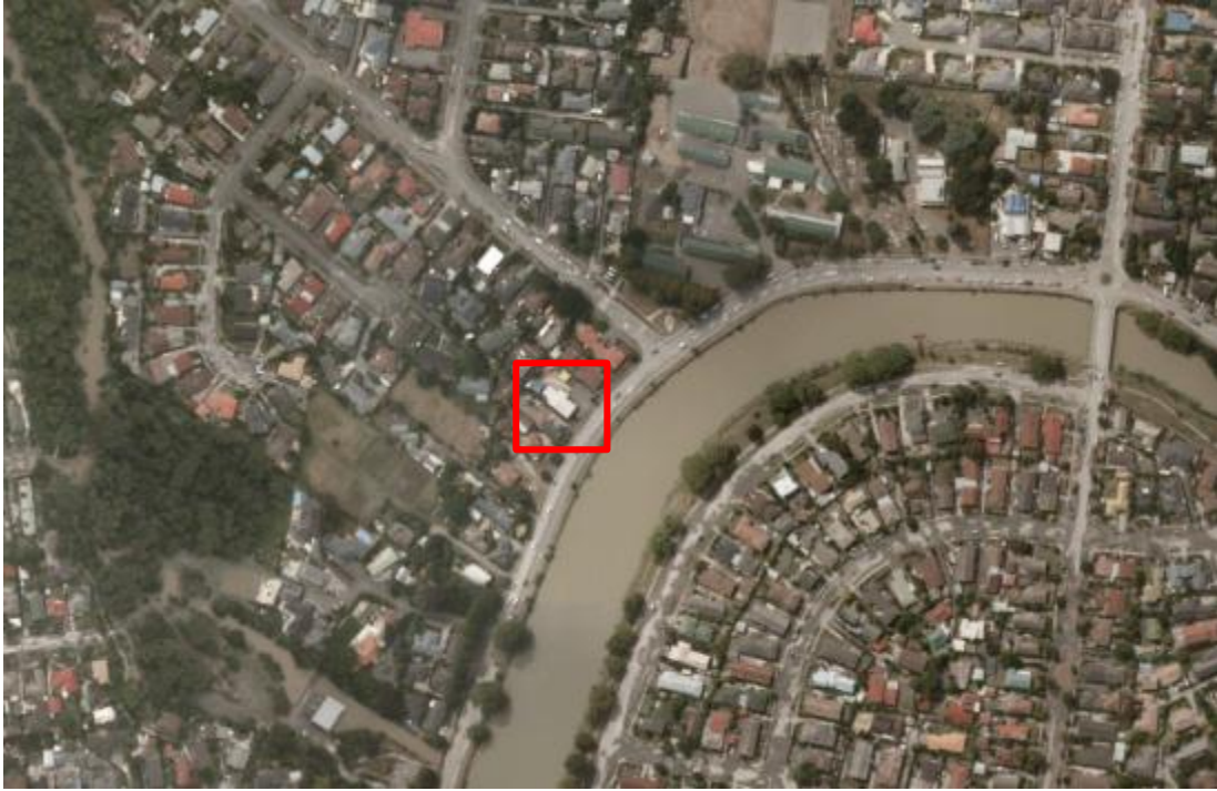
Aerial photo: Liquefaction is visible in the surrounding area.
