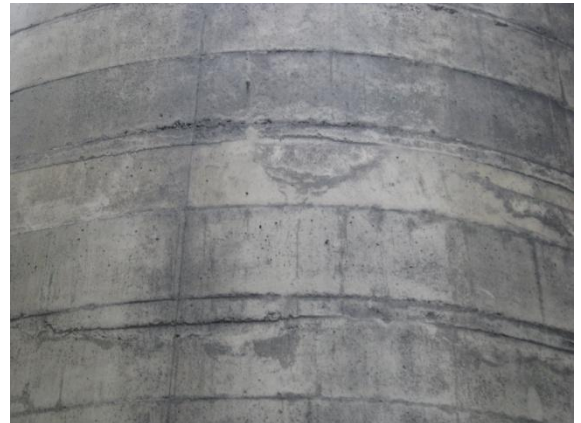
Photo 8: Shuttering marks
