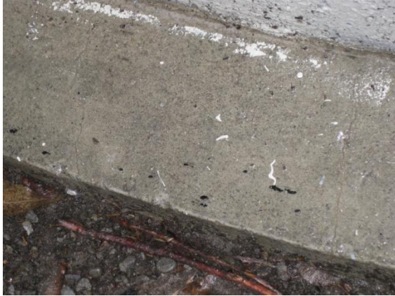
Photo 5: Hairline cracks in top of concrete foundation to the north of the entrance
