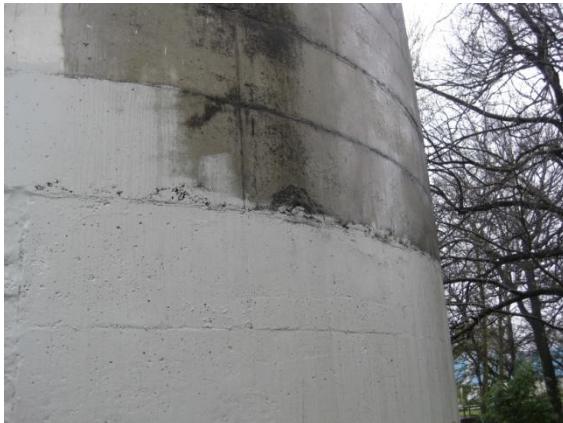
Photo 7: 450mm high shuttering marks in concrete wall.
