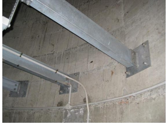
Photo 18: Steel beams for telecommunications equipment anchored to the concrete wall
