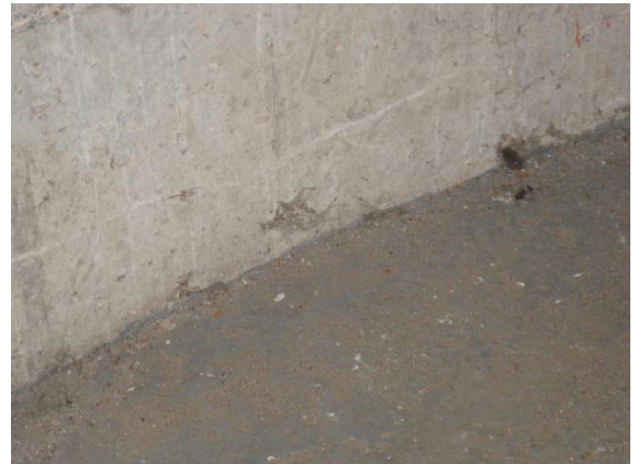
Photo 16: Joint between the concrete foundation and concrete wall
