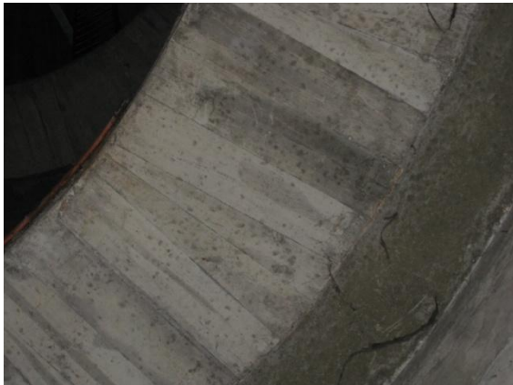
Photo 15: Joint between 850mm wide concrete ledge and concrete wall
