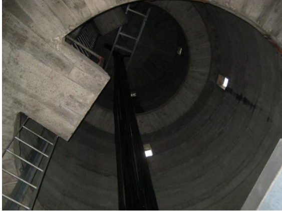
Photo 13: Interior of tower from ground level showing the 850mm wide ledges and ladders
