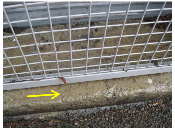
Photo 4: Hairline crack located at entrance in top of concrete foundation
