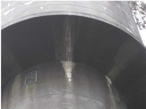
Photo 19: Build up of calcium carbonate noted on the underside of the top level extension indicating water leakage.
