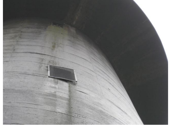
Photo 10: Grated openings (4 per level)
