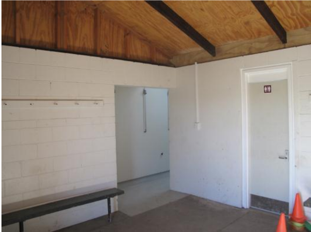
Photograph 5 Concrete masonry lintel over openings
