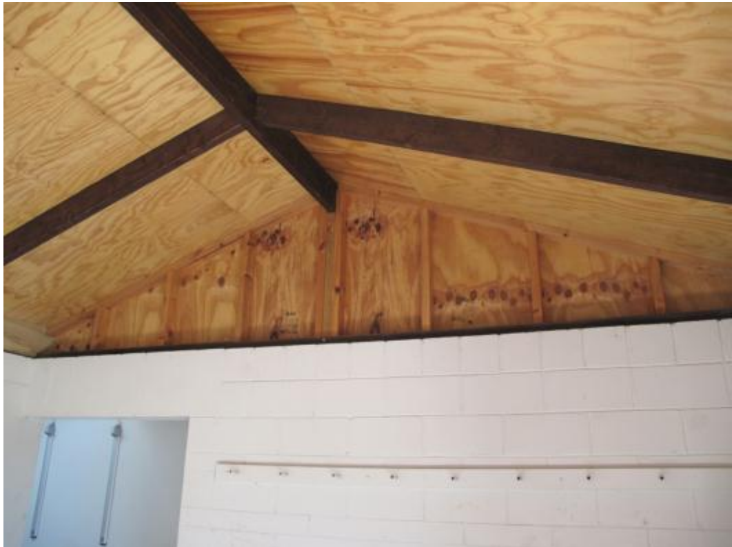
Photograph 6 Plywood lined timber roof structure
