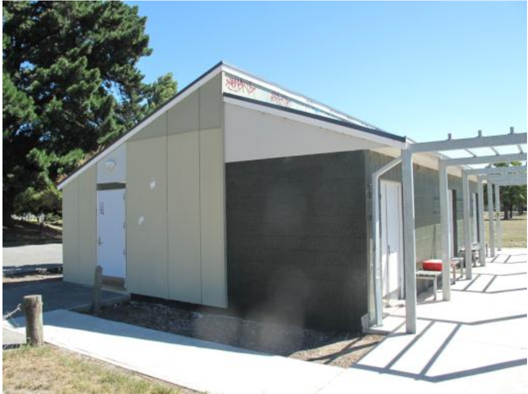
Photograph 3 Eastern elevation of the building
