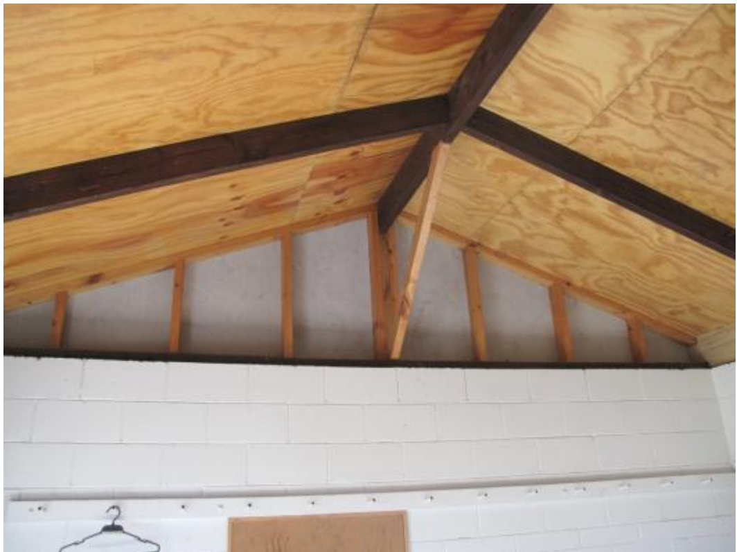
Photograph 4 Timber framed infill wall
