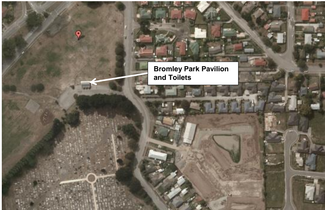
Figure 4 Post February 2011 Earthquake Aerial Photography 3
