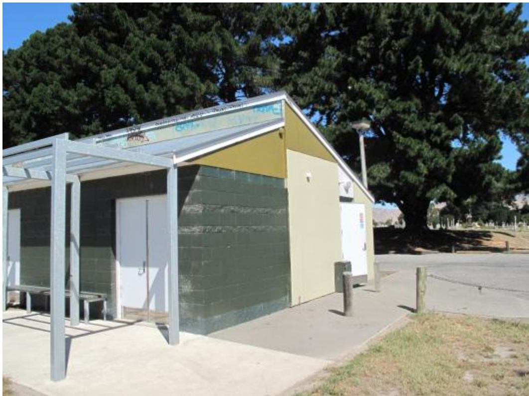
Photograph 2 View of the building from the north-west
