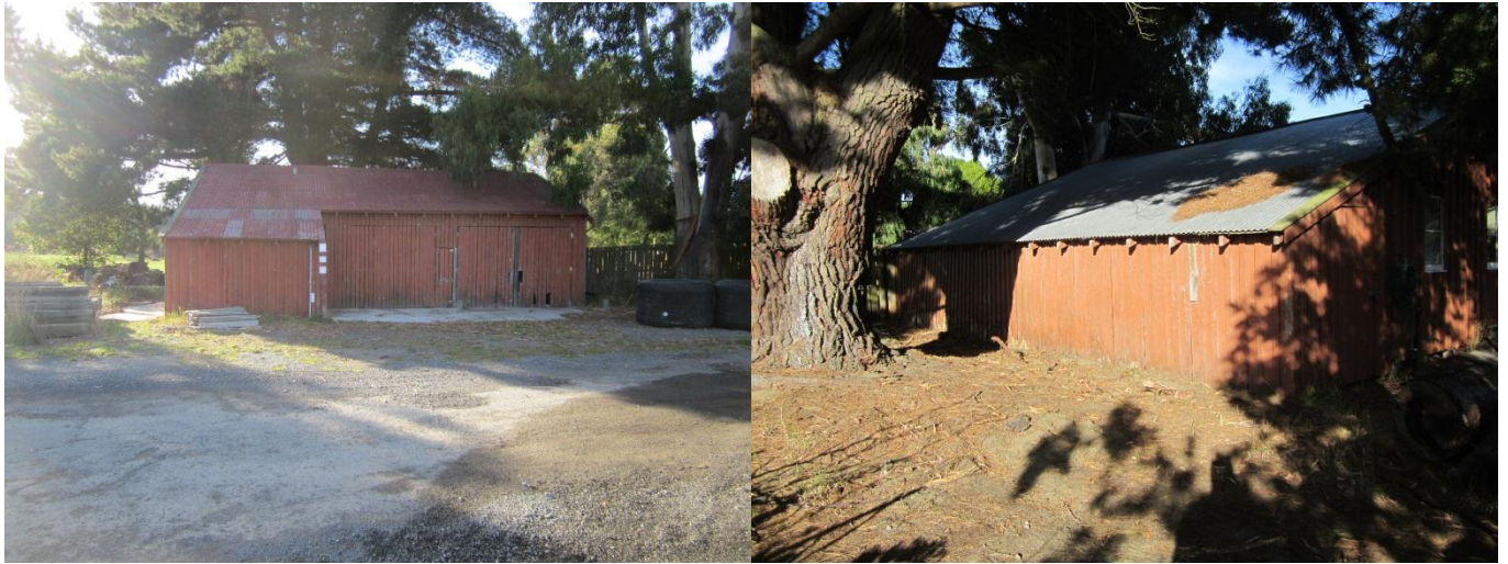
Elevations of the exterior of the old woolshed
