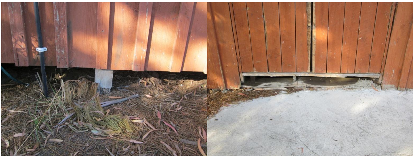
Photos showing a timber floor founded upon timber piles and bearers
