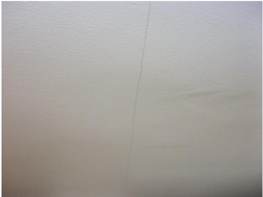
Photograph 7: Minor cracking in plasterboard
