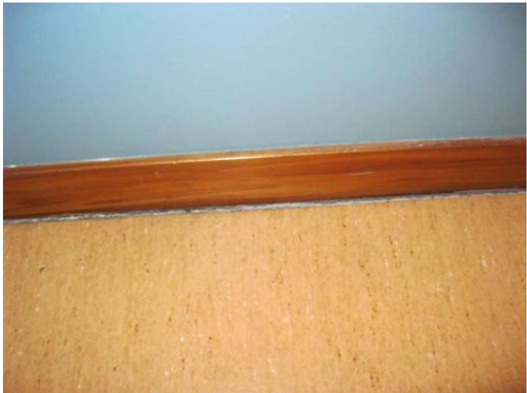
Photograph 6: Separation between concrete floor slab and timber framed wall
