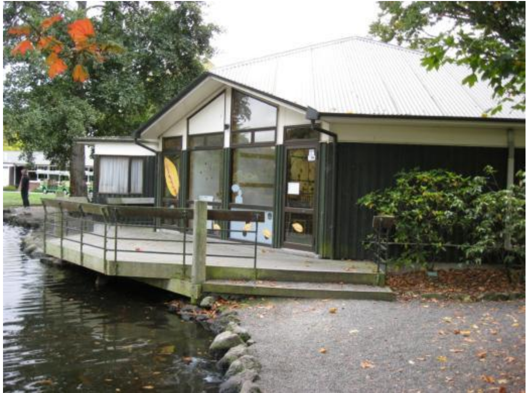
Photograph 3: Balcony and structure abutting lake with insignificant short column potential
