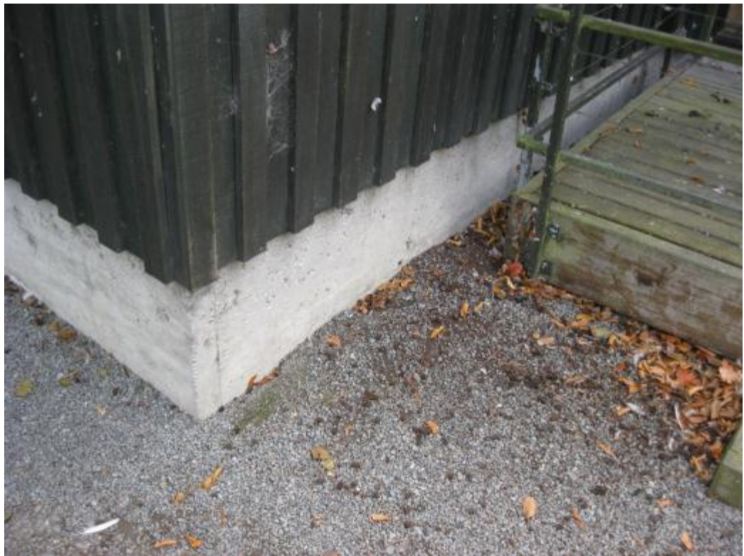
Photograph 4: Perimeter strip footing supporting timber framed walls
