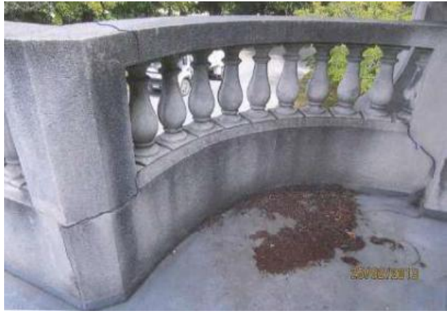
BALCONY CRACKING
