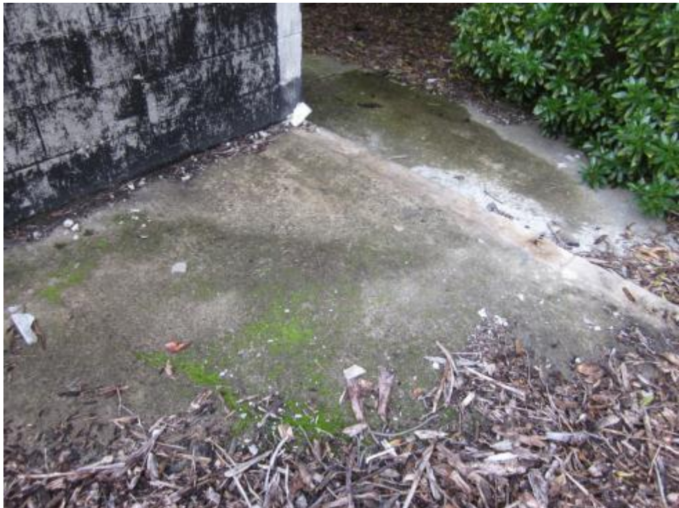
Photograph 6: Leftover concrete pad and southern external wall.
