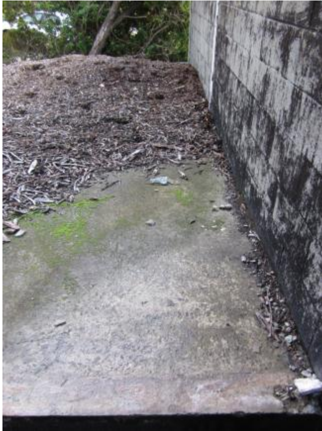
Photograph 7: Leftover external concrete pad adjacent to southern external wall.
