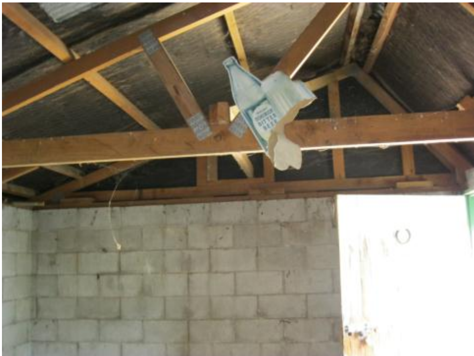
Photograph 10: Interior view of timber trusses and external concrete masonry walls.
