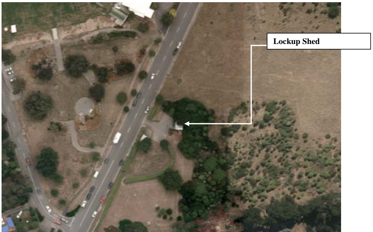
Figure 3 Post February 2011 Earthquake Aerial Photography 2
