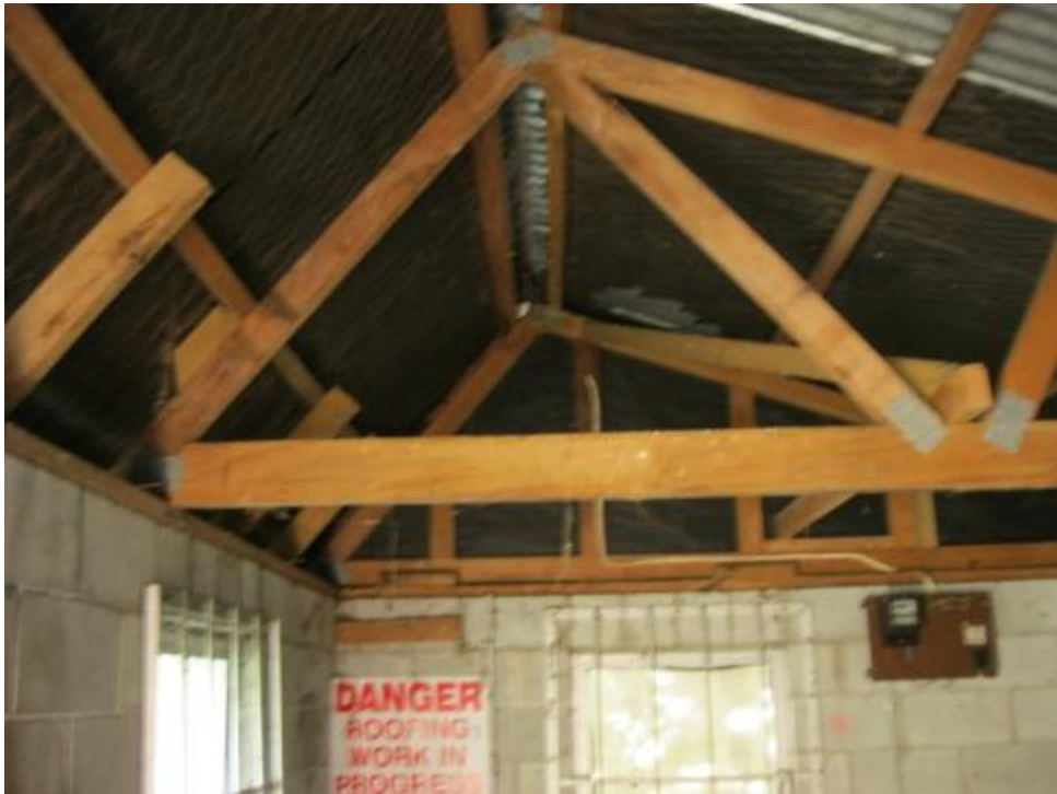
Photograph 9: Interior view of timber roof trusses and external concrete masonry walls.
