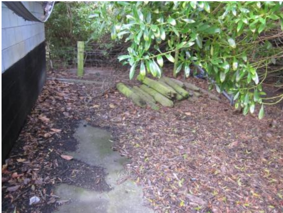
Photograph 8: Concrete pad at eastern side of structure used for timber storage.
