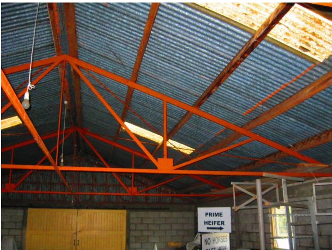
Photograph 6 Steel roof cross bracing visible in roof space
