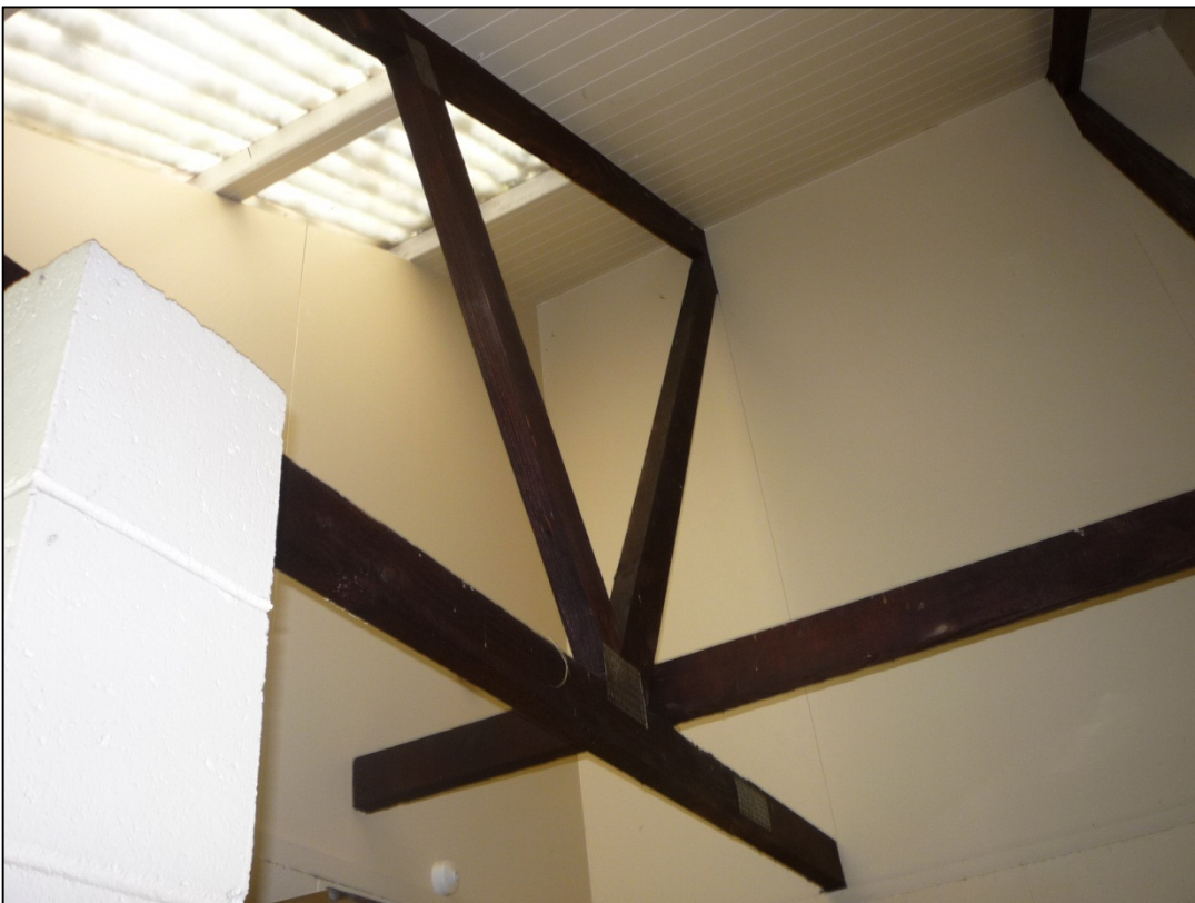
Photo 4: Typical view of roof truss. Note no ceiling diaphragm.
