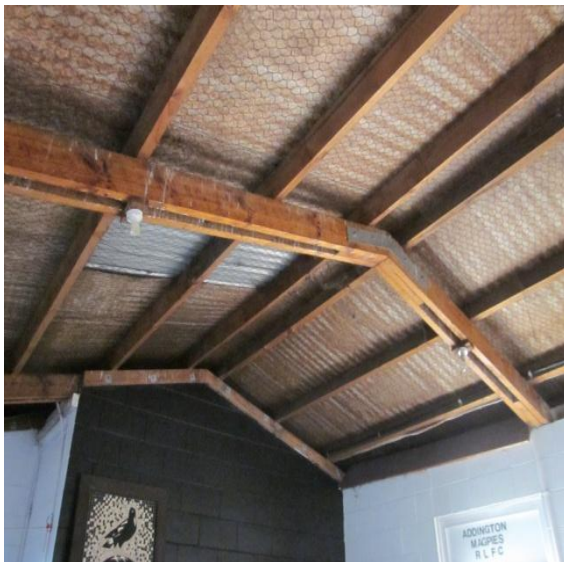
Photo 3: Interior of the roof showing typical roof framing
