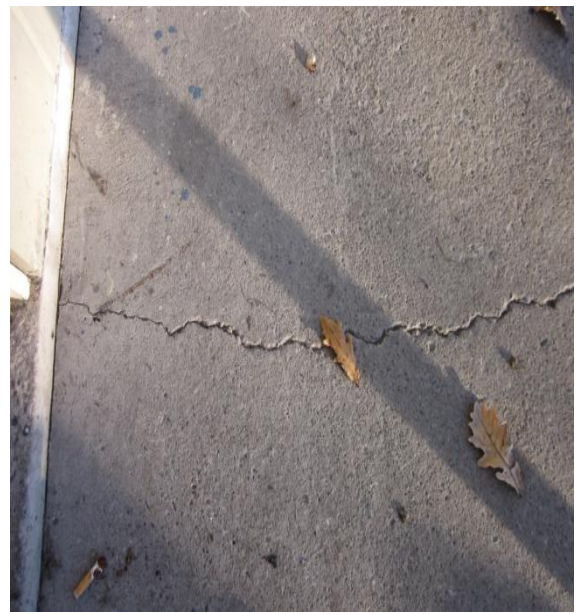
Photo 6: Detail of existing cracking in the external concrete slab which has been exacerbated by the recent earthquakes
