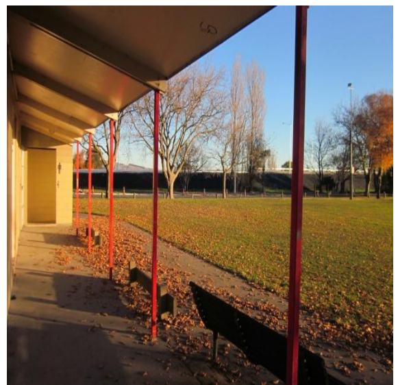
Photo 4: Verandah on the west side of the building where the roof is supported by steel posts
