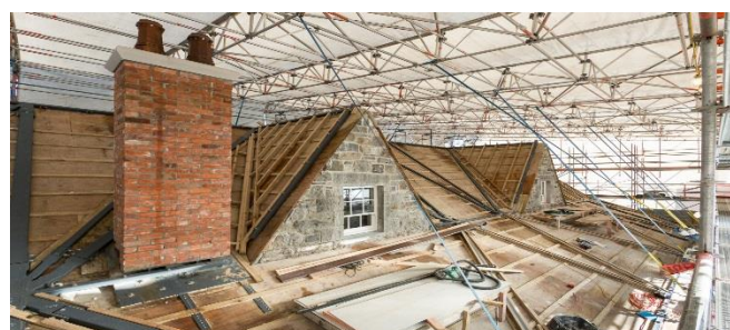
Steel Diaphragm to Roof after installation
