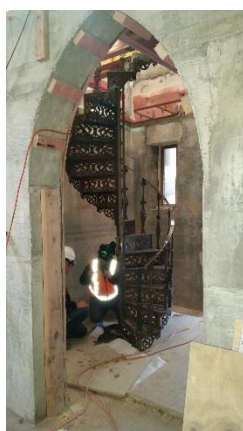
Refurbished spiral staircase
