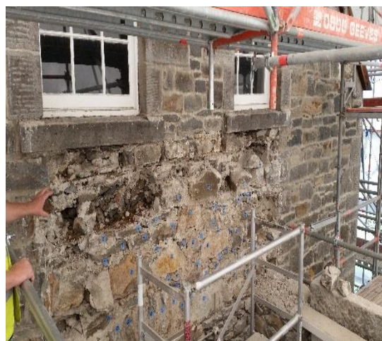
Deteriorated Stone Work to end Gable Walls
