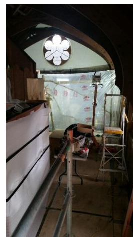
Containment tent at the front of the Chapel for the removal of the Asbestos.
