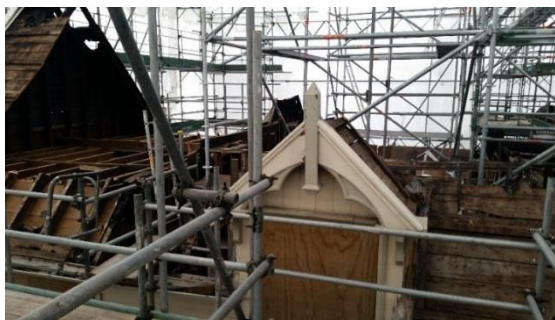
First floor fire damage underneath the scaffolding structure and wrap.
