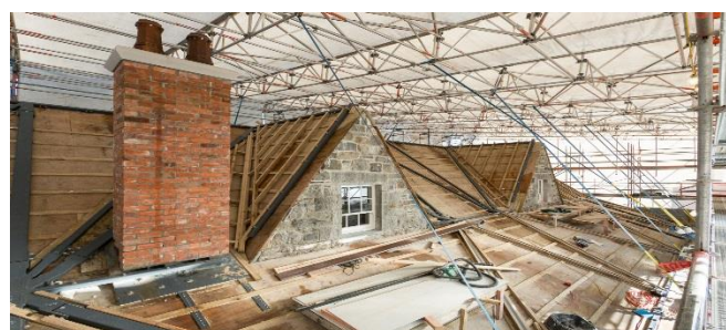
Steel Diaphragm to Roof after installation
