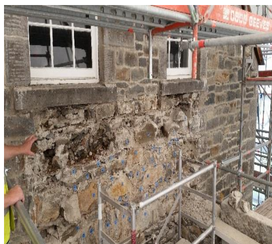
Deteriorated Stone Work to end Gable Walls
