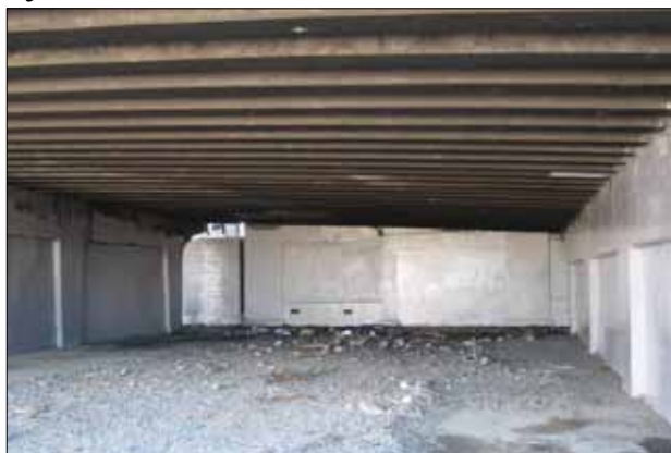
Under the Colombo Street Over-bridge
