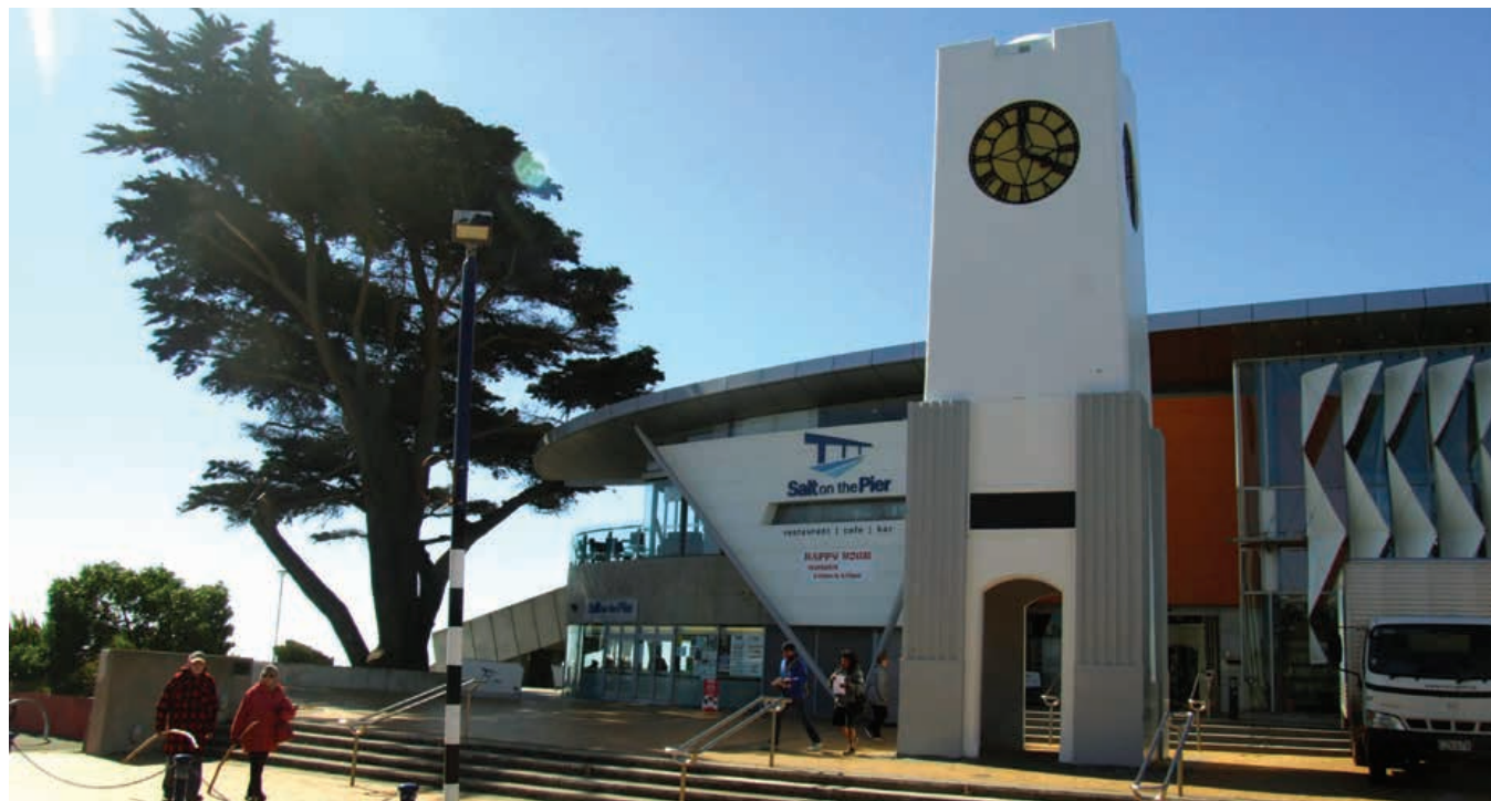
Figure 39: Photograph of the New Brighton Library
