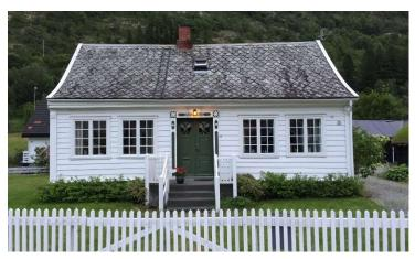
Figure 4 - House in Lærdalsøyri with about 10% glazing to the front wall (including projected area of roof)
