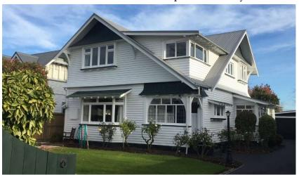
Figure 1 - House in Strowan with about 20% glazing to the front wall
