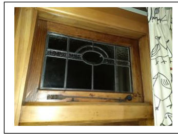
Lead-light double-glazed and original hardware retained.
