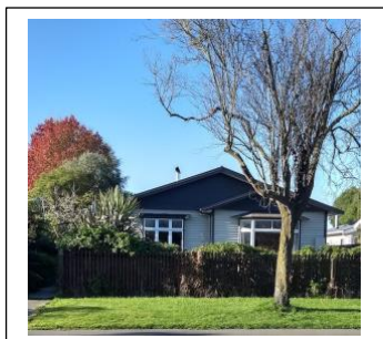
Single storeyed bungalow with weatherboard cladding and low-pitched gable roof with eaves.
