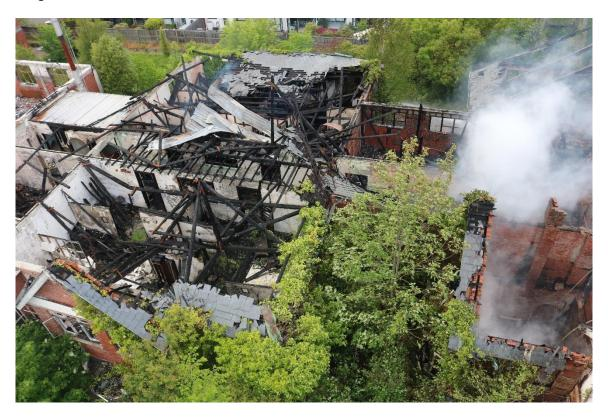
Fire connected at first floor level to previous fire. Total loss of supporting roof structures.
