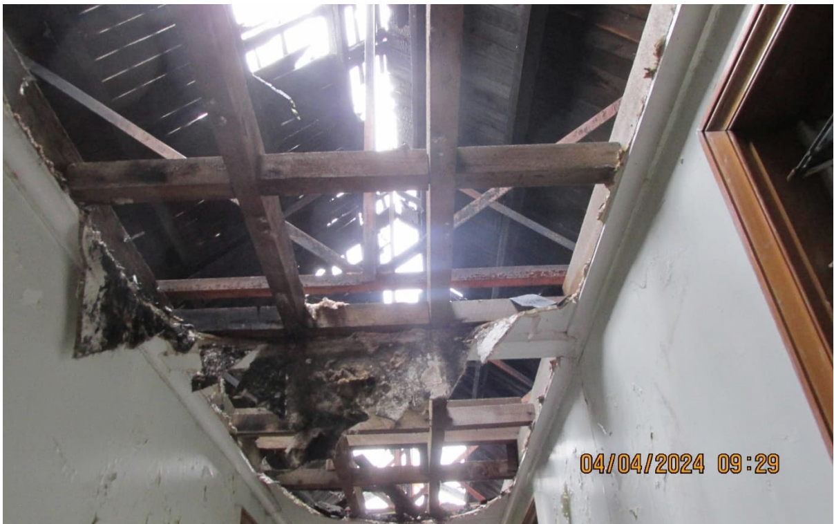
South-East End Roof Structure (fire damage accommodation block)
