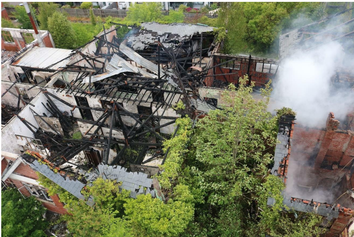
Fire connected at first floor level to previous fire. Total loss of supporting roof structures.
