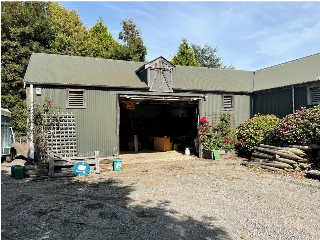
Photograph 22: Image of garage/hobby workshop. Image taken facing south-west.
