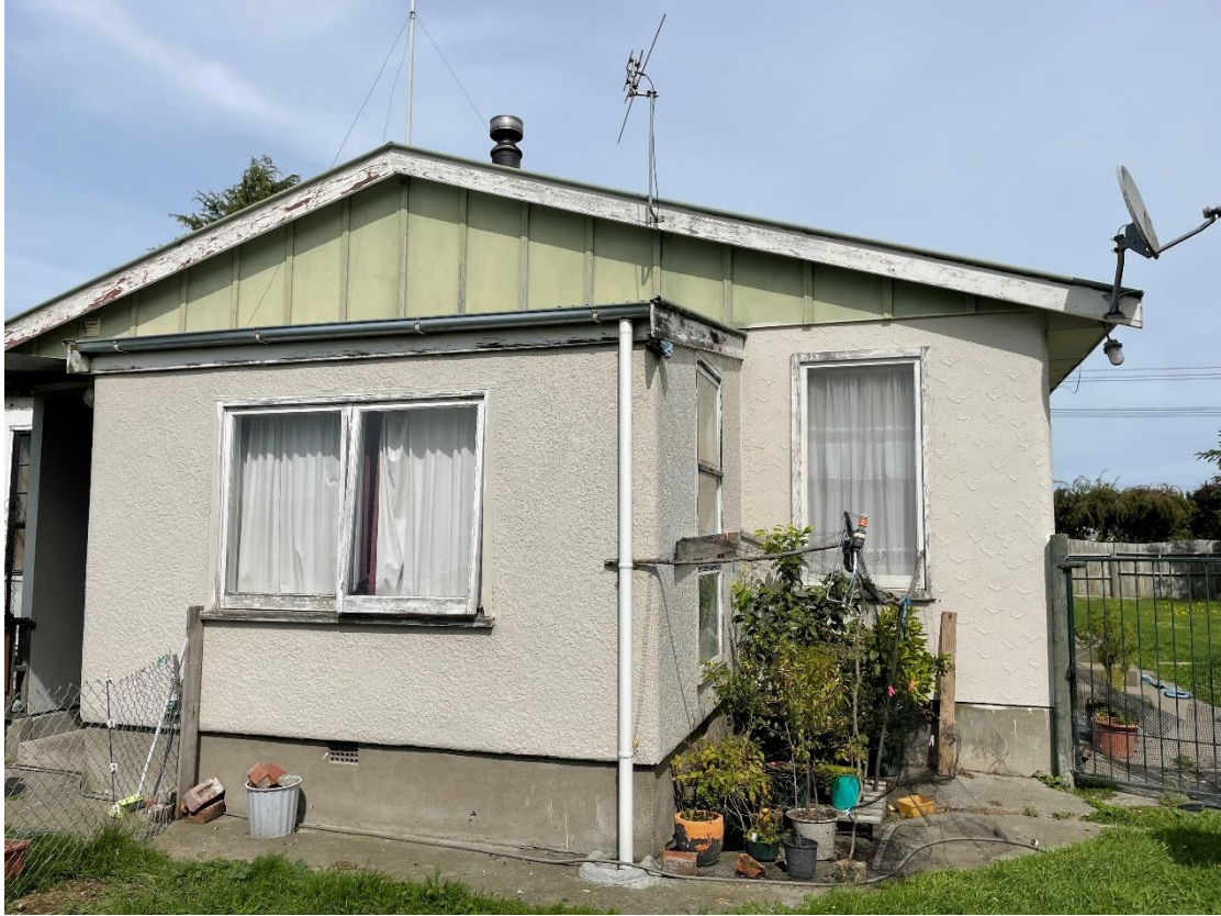
Photograph 27: Image of dwelling at 27 Marshs Road. Image taken facing south-west.
