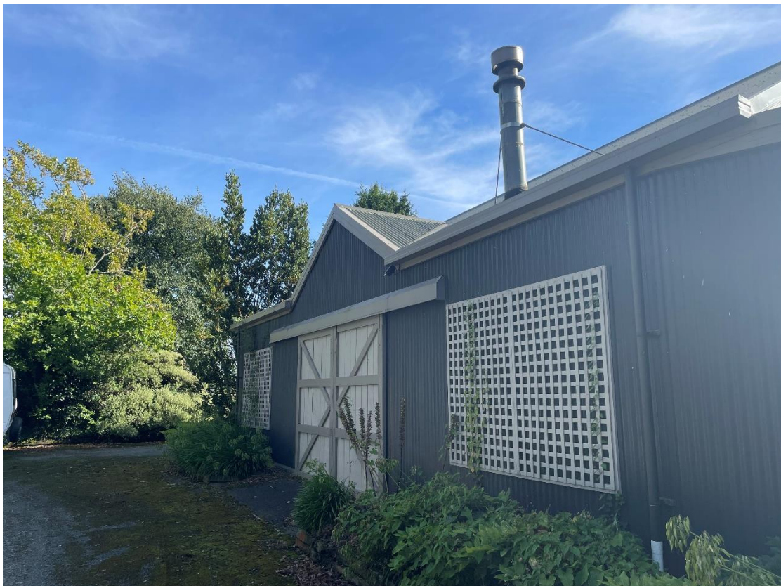
Photograph 10: Front of garage. Image taken facing north-west.
