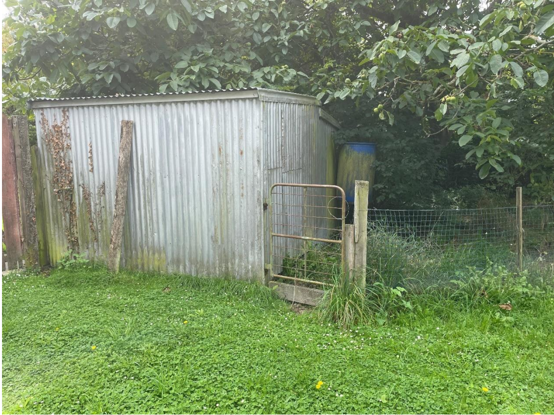
Photograph 38: Storage shed, image taken facing north-east.
