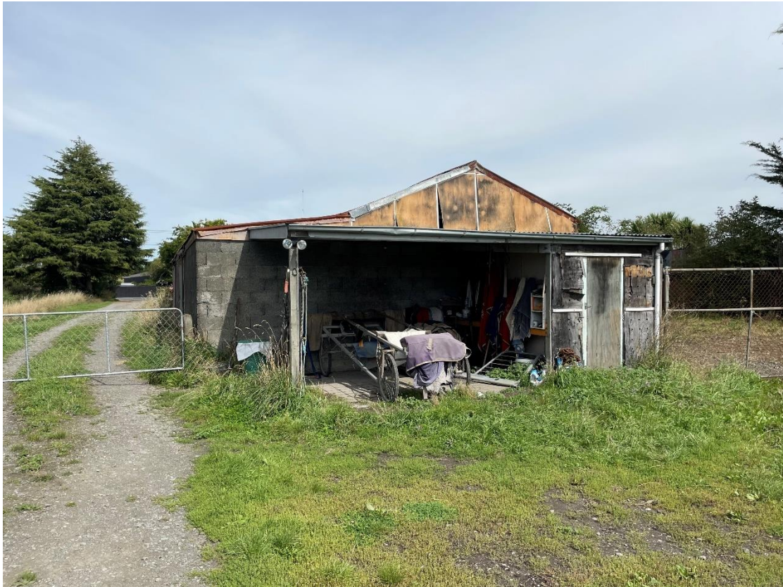
Photograph 32: Image of storage shed. Image taken facing south-west.
