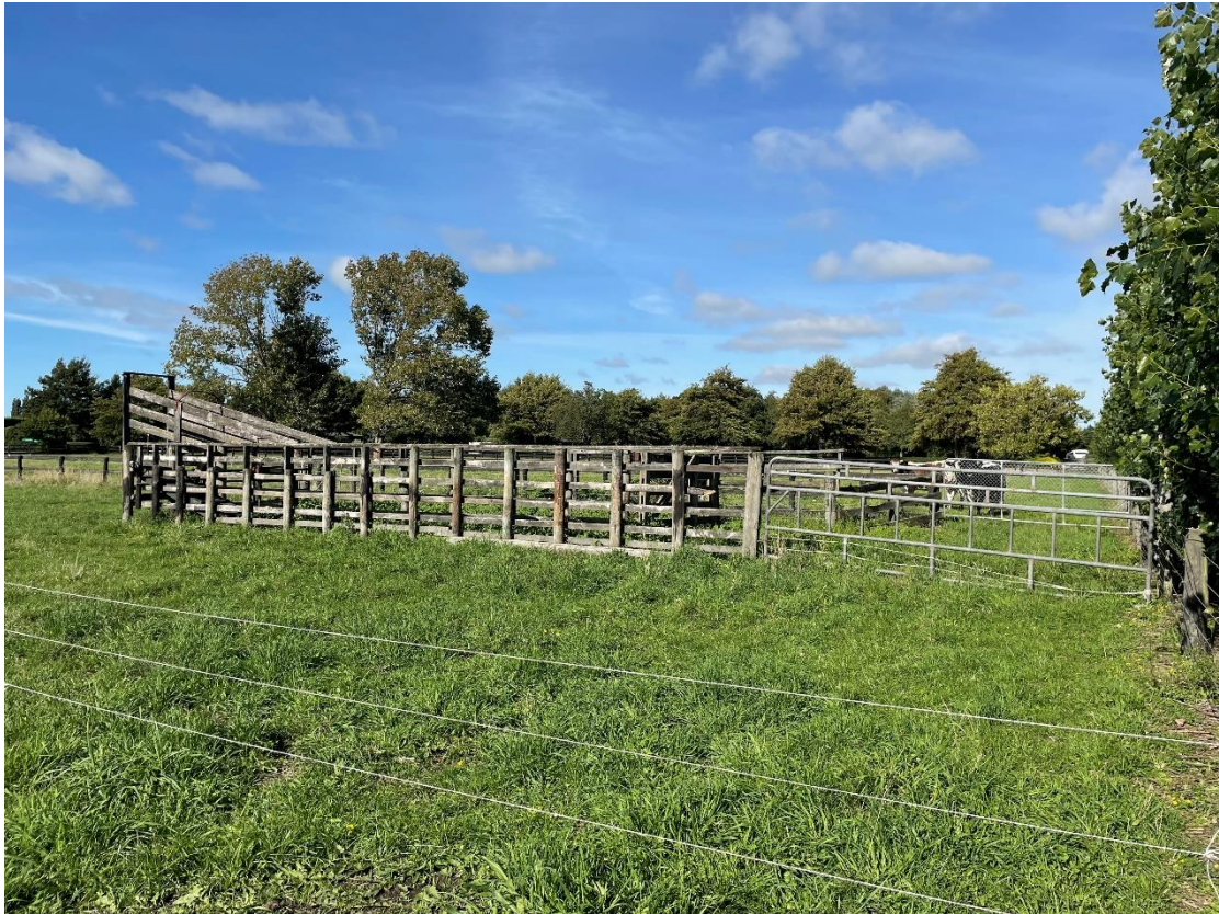
Photograph 15: Stock loading ramp.
