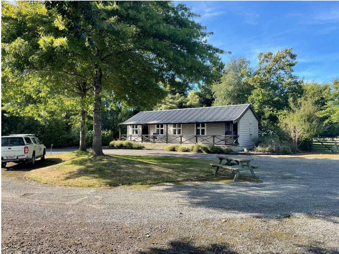
Photograph 5: Cottage style building. Image taken facing east.
