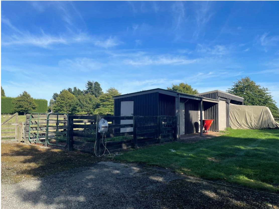
Photograph 1: Storage shed near western paddock. Image taken facing west.
