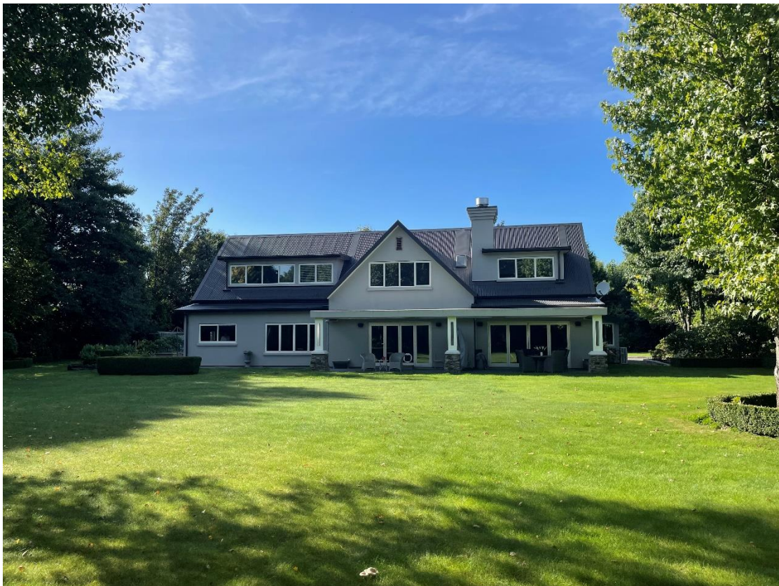
Photograph 6: Main dwelling, image taken facing south-east.
