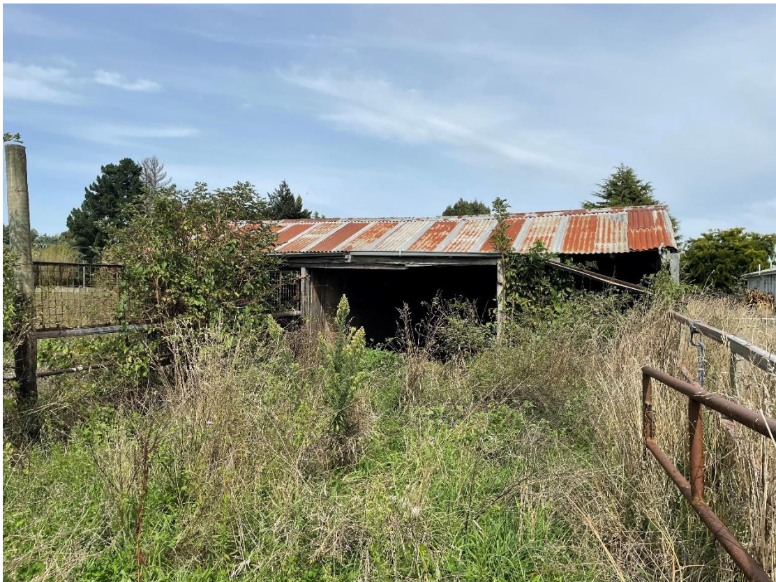
Photograph 31: Image of derelict horse stables. Image taken facing south-west.
