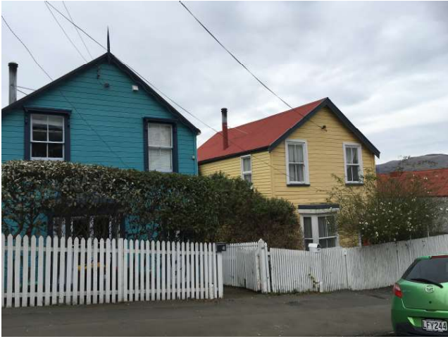
EXAMPLE 1: Steep gable roofs, variety of paint colours, with horizontal weatherboards and medium-sized vertical windows.
