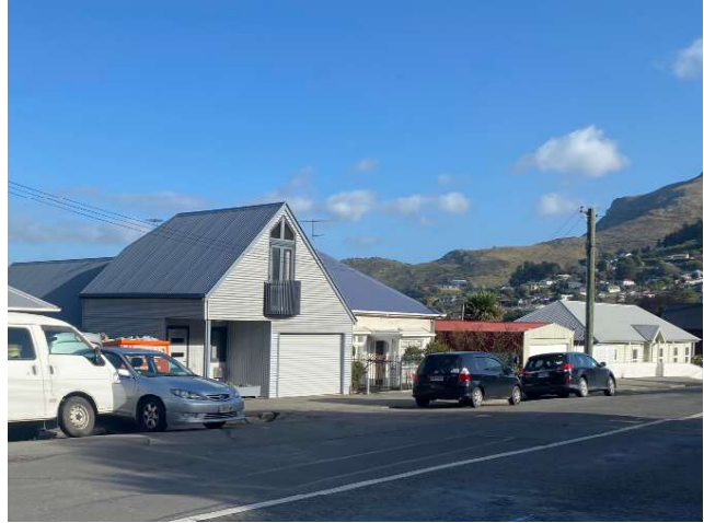
EXAMPLE 8: Corrugated iron is used as the primary or sole cladding material. This material is not considered representative of a 'Primary' attribute.
