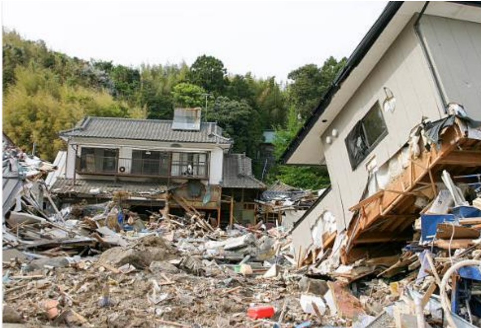
Figure 10. Tsunami damage in Murohama Miyato, Japan 2011, iStock by Getty Images
