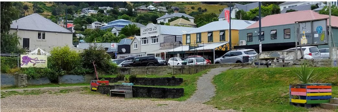
Figure 4: London Street viewed from the south east (cnr of London and Oxford Street, including heritage buildings)
