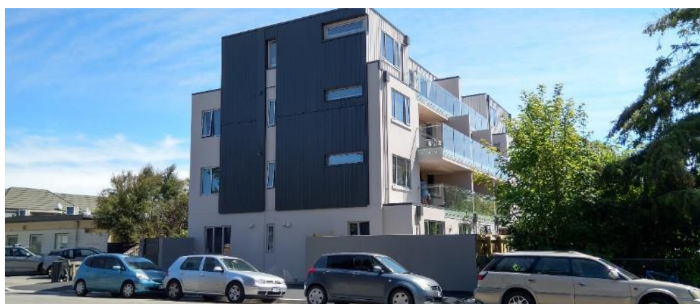
Four storey development built lengthways on a narrow section creates issues of overlooking and enclosure for neighbours
