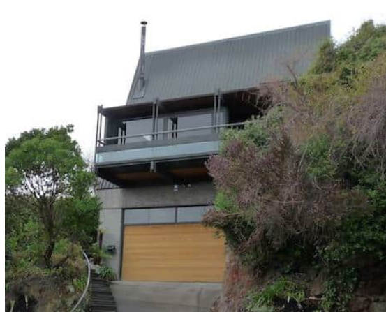
The former Hardie house.
