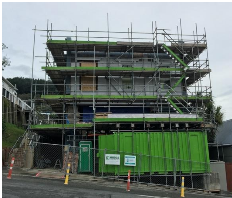
Former Kilwinning Lodge, Canterbury Street, under repair. Dr A McEwan, July 2021.
