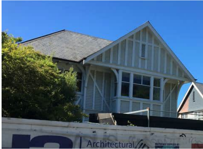
The former home of Sir Hamish and Lady Hay, 70 Heaton Street. Dr A McEwan
