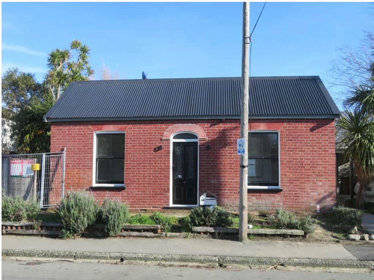
5 Shelley Street after seismic strengthening and conservation. T Ussher, CCC Heritage Files, 14 July 2021.
