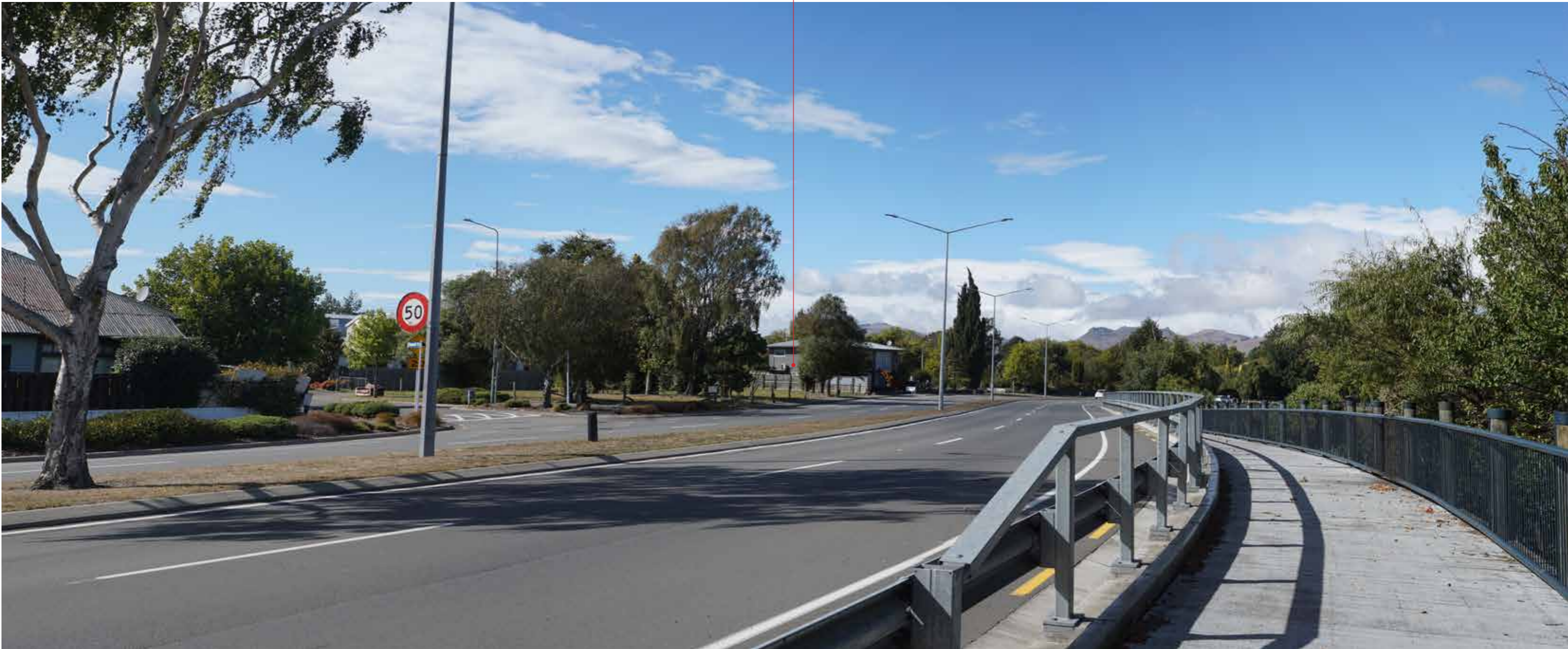
A. EXISTING VIEW
