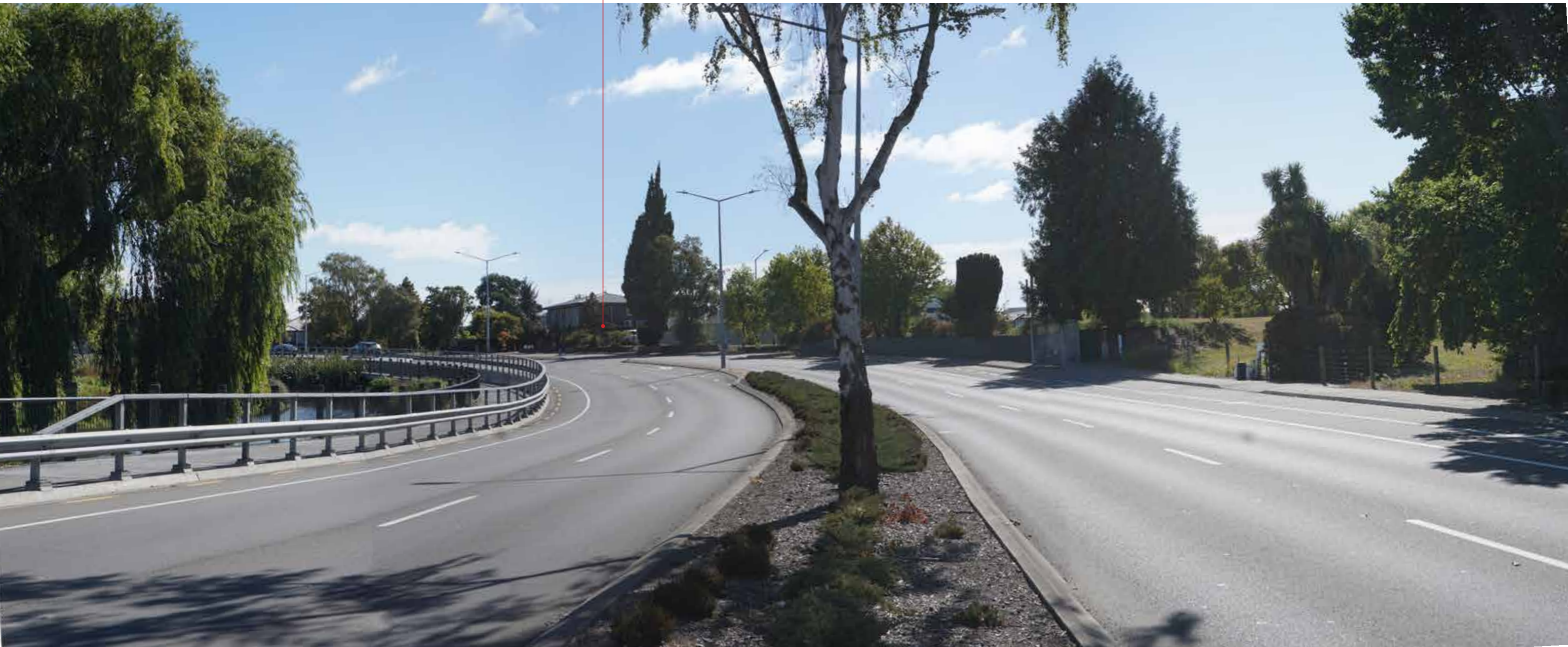
A. EXISTING VIEW
