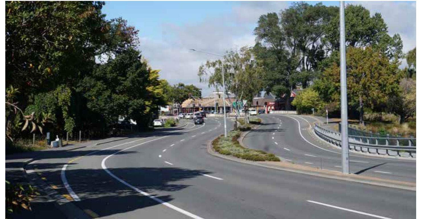
D Fitzgerald Avenue is the main north - south connection along the eastern boundary of the city centre, carrying large volumes of traffic in both directions with a dual carriageway, on-road cycle paths and footpaths on both sides.. The road forms a significant barrier or corridor between the Ōtākaro-Avon River and the proposal site.
