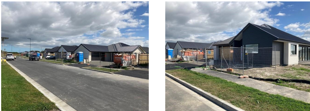
Figure 6: Site Photos – Gisele Crescent under Construction – Single storey standalone houses
