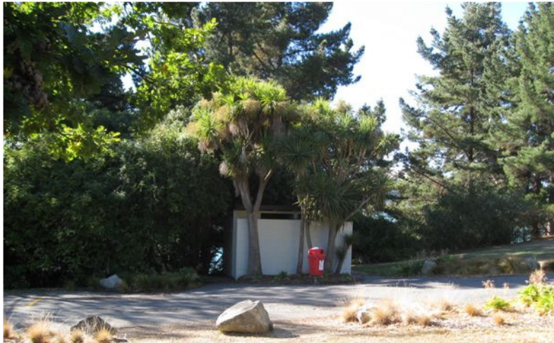
Stoddart Point picnic area toilet block, hidden by surrounding vegetation. Photo taken in April 2010.
