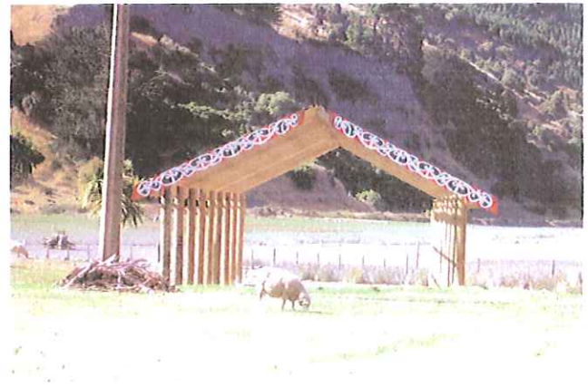
Figure 12: Te Wharewaka under construction
