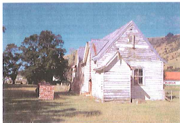
Figure 10: The Old School Building
