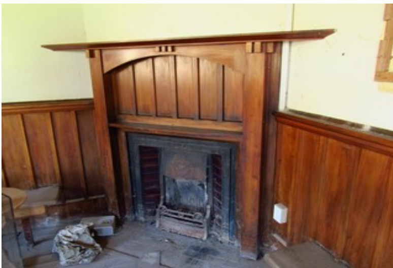
Source: B.Dougan 31/3/2015 Coal register fireplace in Reading room flanked by glazed tiles and Rimu surround. Note intrusive surface mounted power outlet.
