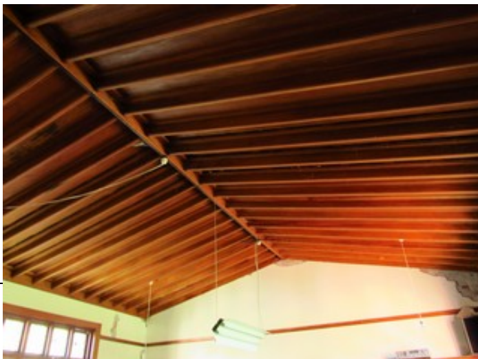
Source: B.Dougan 31/3/2015 The ceiling of the Library Room in the Arts and Crafts style. The ceiling is unusual, being suspended below and independently of the roof structure, and in the detailing and incorporation of the ceiling vents.
