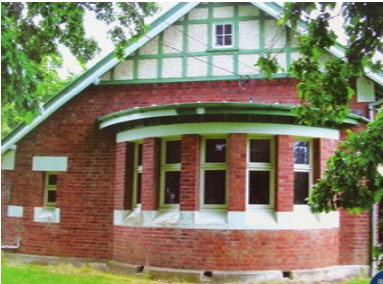
Source: Akaroa Mail 2010 Bay window to the east elevation articulated as a separate building element with a flat independent roof. Note the stippled plaster gable and /high-level fixed non-operative fanlight.
