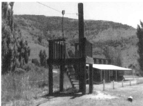
Figure 5: The beginning of the flying fox, the community hall is in the background
