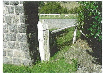
Original timber post and fence
