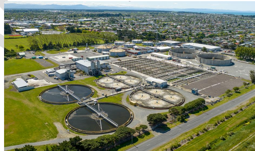
Christchurch Wastewater Treatment Plant.
