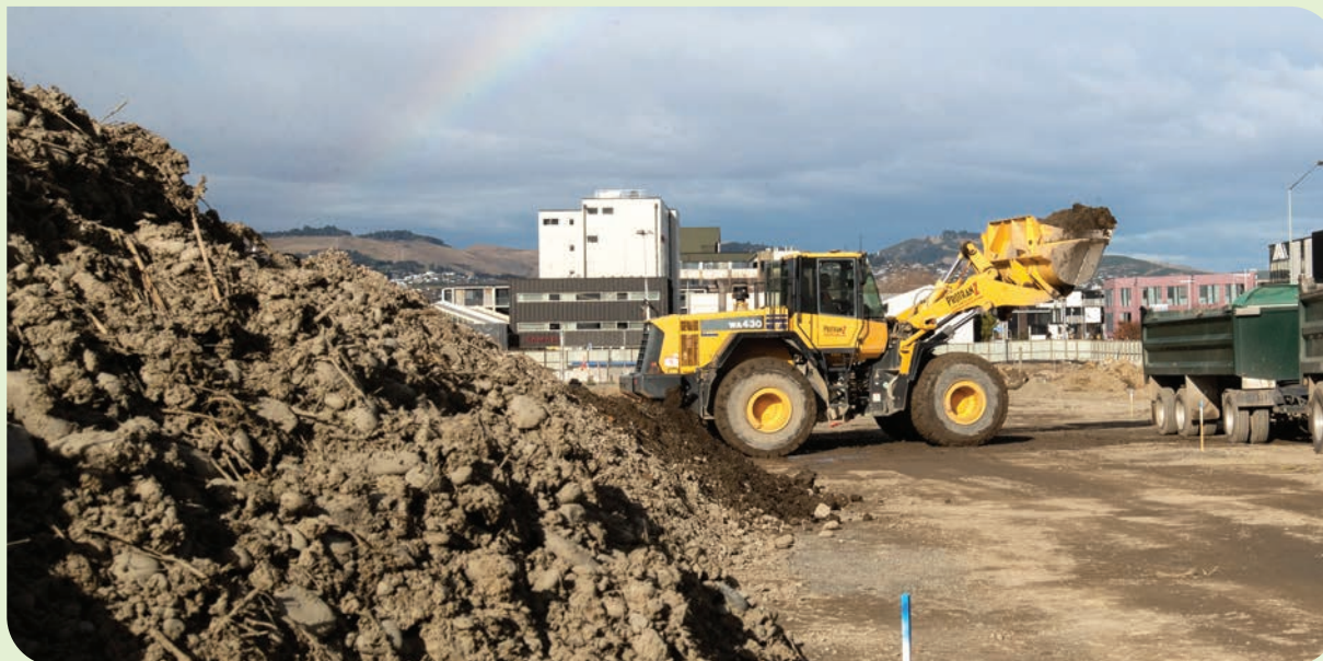
Early works, July 2019.
