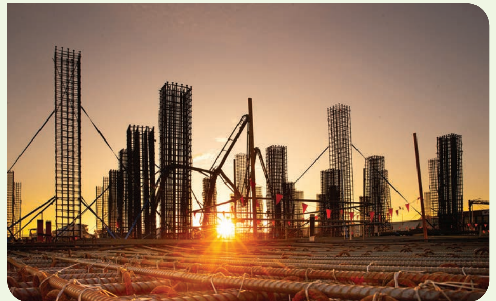
Concrete pour, January 2023.
