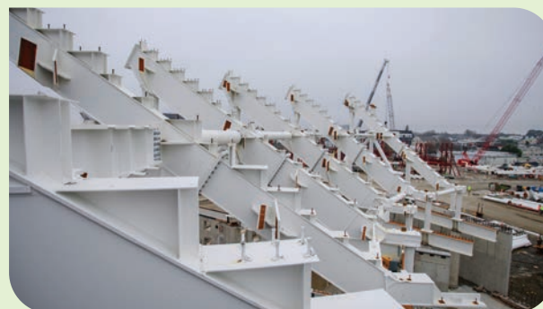
Prefabricated steel work being installed in the northwest stand, July 2024.
