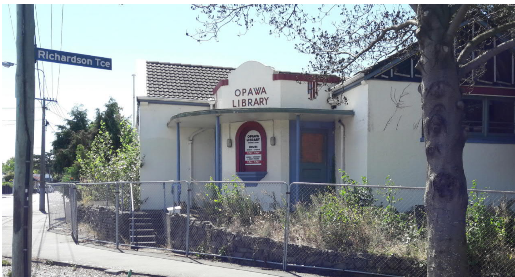
Existing front entrance
