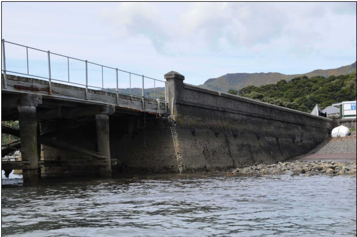
Photo 24 The junction of the abutment, and its concrete wall, and the start of the timber wharf structure on the south side. Galvanised steel railings have replaced the painted timber railings since 1973.
