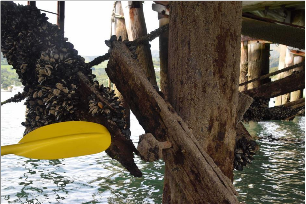
Photo 33 Broken timber brace.
