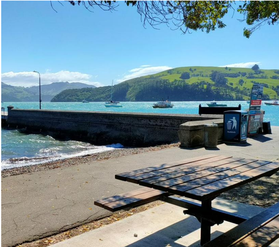
Figure 66. View of south elevation of the concrete abutment of the Akaroa Main Wharf. Visible in the image is the main concrete portion topped by concrete parapet wall. Image also shows an associated protective concrete wall running a short distance along the foreshore atop the sea wall. The image is taken looking northwest. Source: SIA 2021.
