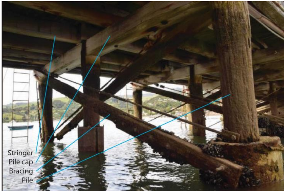
Figure 74. Another example of a 'bent' – the entire frame comprising, this time, three piles with a capping beam on top and bracing to provide rigidity (Origin 2019).
