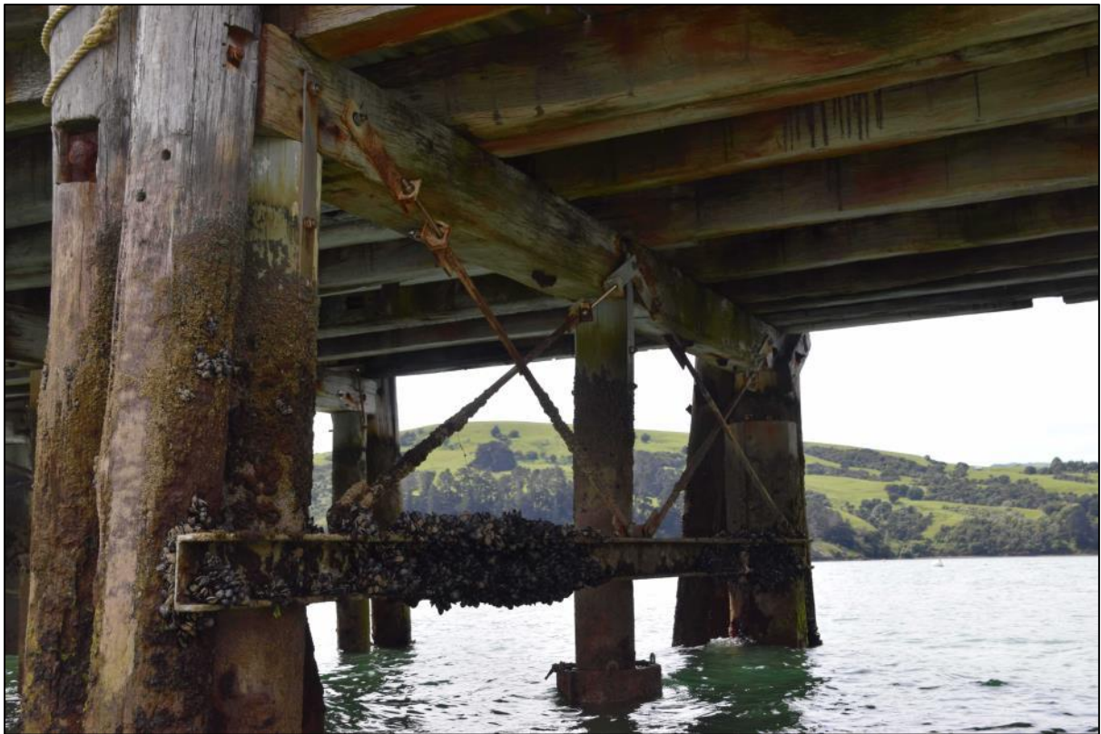
Photo 30 An example of modern steel repairs – bolted straps between the piles and cap beam, a steel PFC horizontal tie and double steel bracing rods. There is also an earlier steel jacket repair to the central pile.
