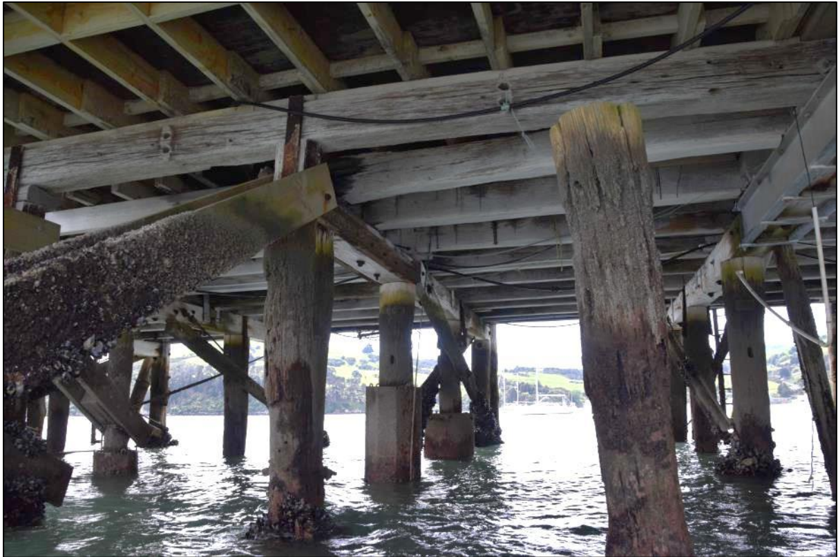
Photo 16 An image underneath the western end of the sheds showing the modern tanalised floor structure to one of the sheds (top) and steel strengthening added to the pile caps (centre and right foreground).
