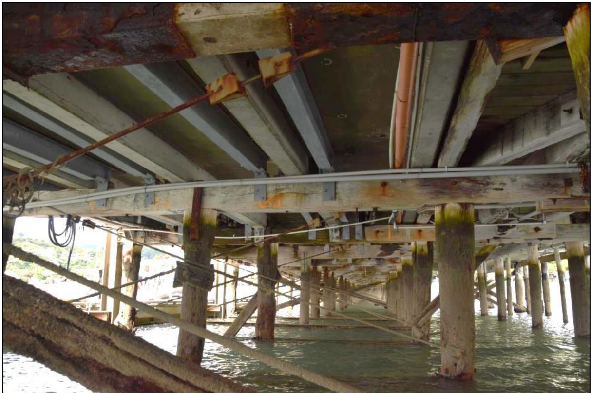
Photo 40 Substantial alterations/repairs with steel and concrete beams below the deck adjacent to the north floating pontoon.
