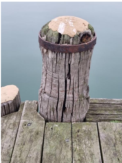
Figure 80. Mooring pile with iron band. Source: South Island Archaeology 2024.
