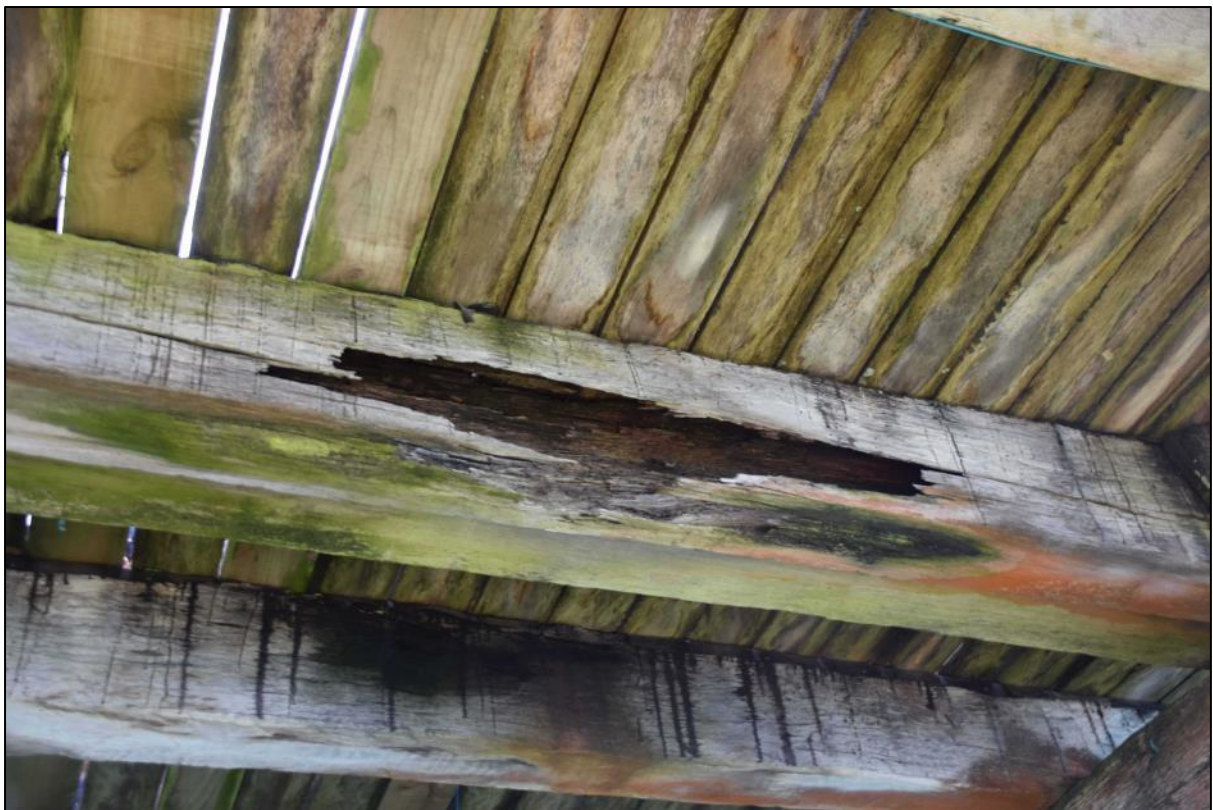
Photo 31 A large area of decay in one of the stringers close to the modern steps toward the western end of the wharf.
