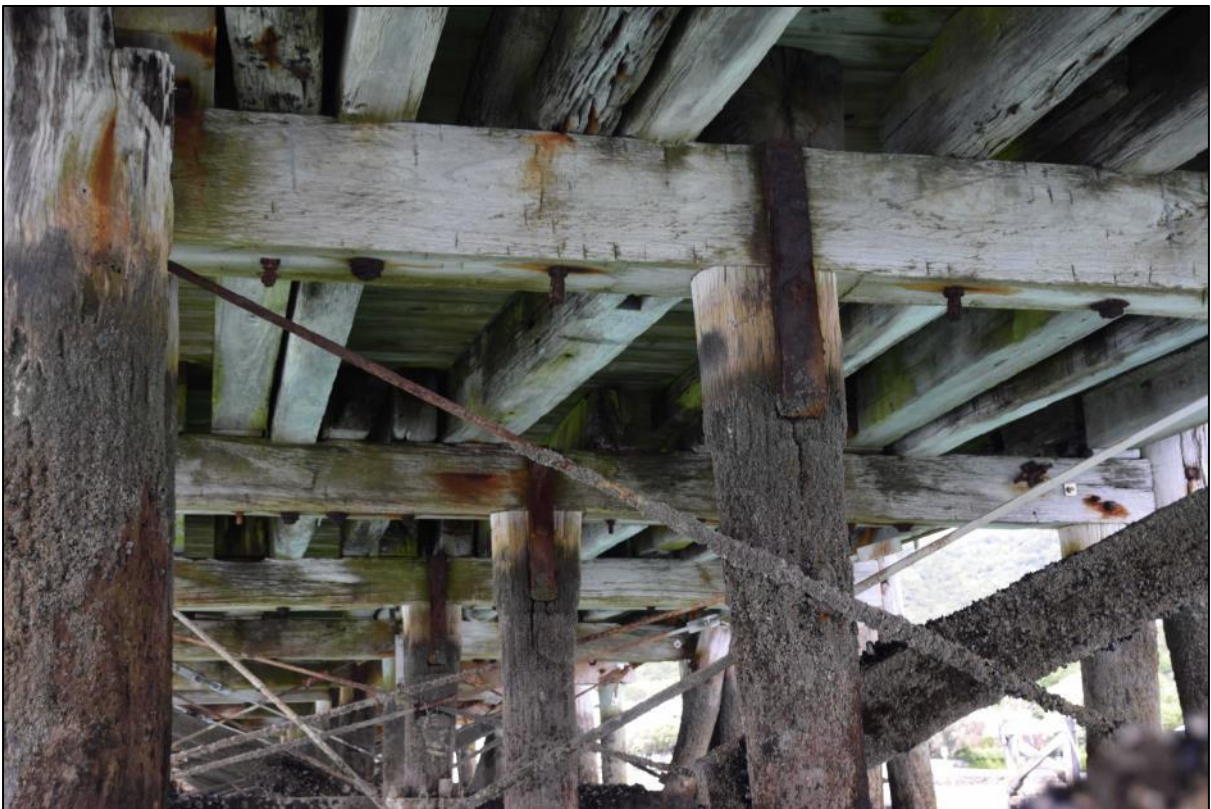
Figure 84. Original wrought iron strap connections between the central piles and their pile cap. The joints also have a mortise and tenon (Origin 2021).
