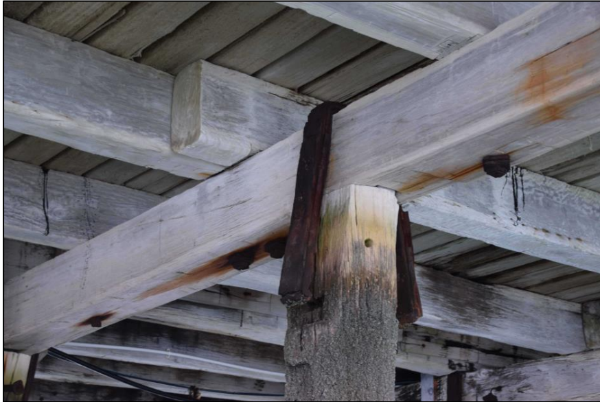
Figure 81. Close-up of the pile head showing the original wrought iron strap connection with the pile cap beam – now corroding/delaminating and separated from the pile head (Origin 2021).
