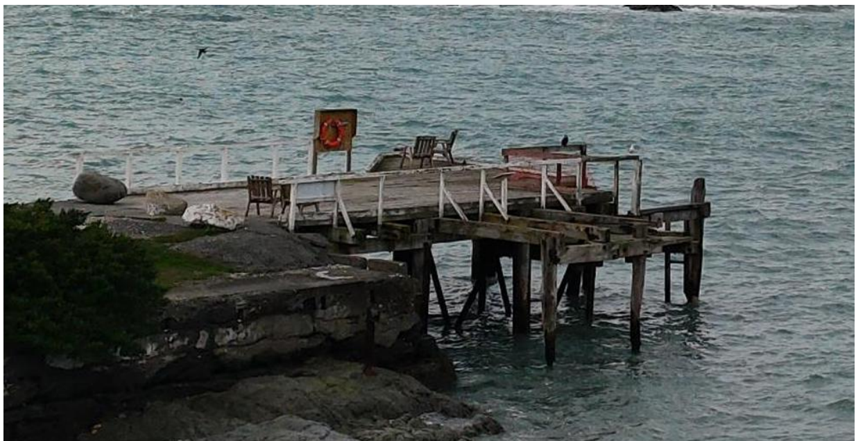
Figure 59. View of westerly side timber jetty that projects from the end of the Old Kaikoura Wharf. Visible in the image are timber piles supporting timber bearers with timber joists running over them. The timber joists are topped by timber deck with deck planking and guardrails. Image taken looking eastward. Source: SIA 2023.
