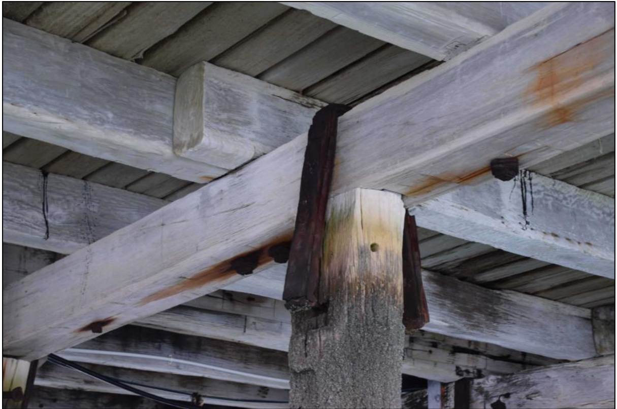
Photo 18 Close-up of the pile head on the right of Photo 17 showing the original wrought iron strap connection with the pile cap beam – now corroding/delaminating and separated from the pile head.
