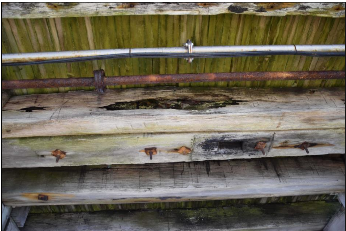
Photo 5 Clear evidence of decay in a timber stringer at the eastern end of the wharf.
