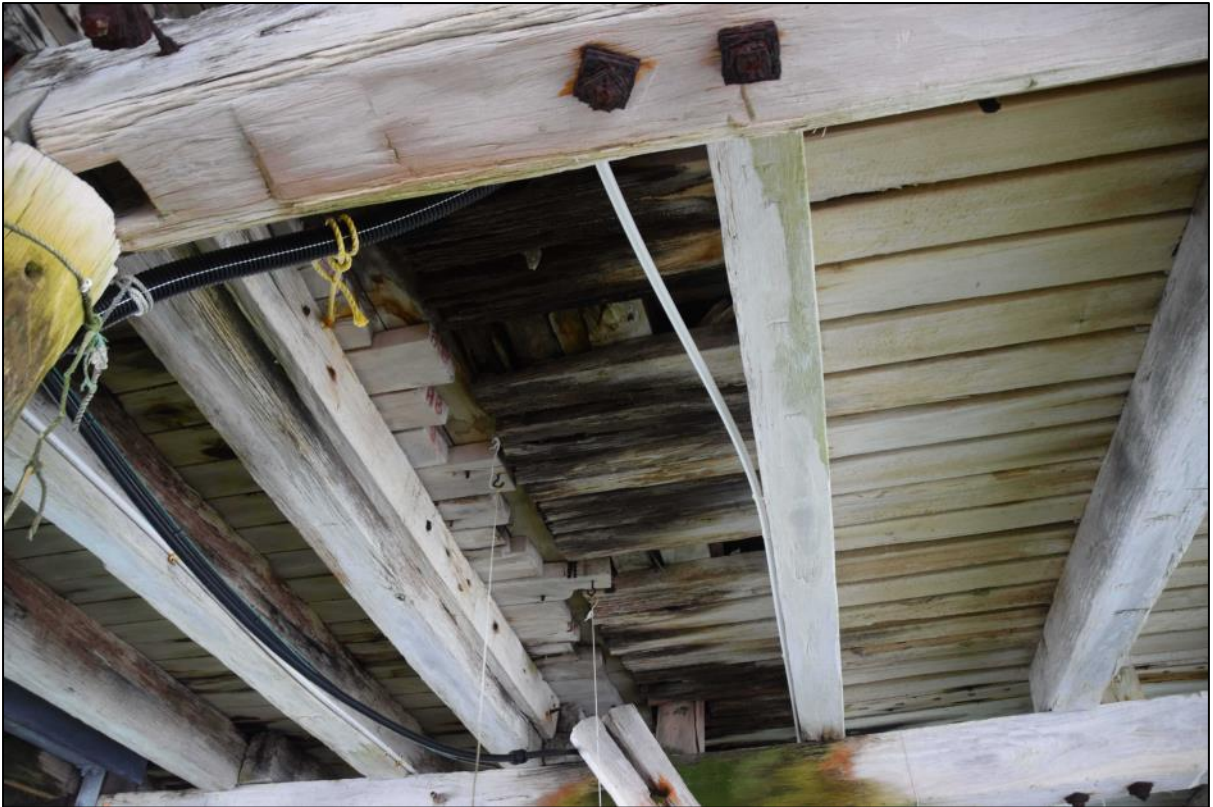
Photo 36 Decay in decking boards beneath the existing deck finish. Corrosion to original iron bolts and nuts.
