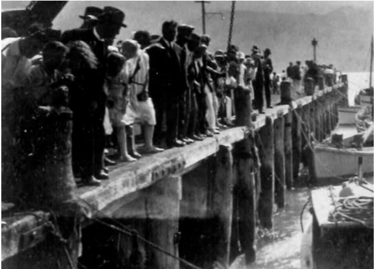
Figure 31. Detail of an undated early 20 th century image showing the iron slice straps on the side of the wharf. Source: Canterbury University Archives.
