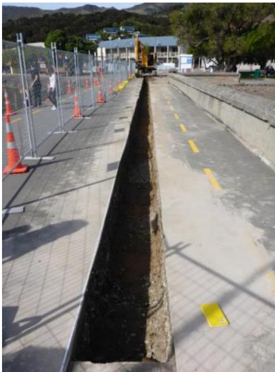
Figure 47. View looking east showing the trench excavated through the solid portion of the Akaroa Main Wharf in 2015 (K. Bennett)
