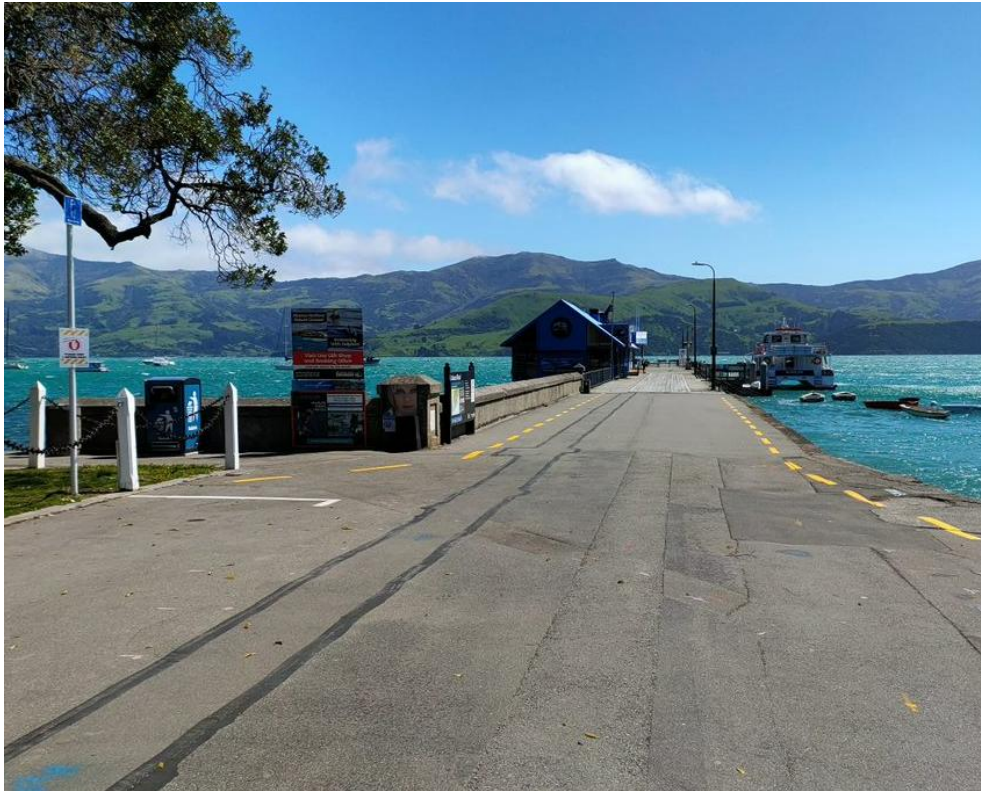
Figure 64. View of concrete abutment portion of Akaroa Main Wharf taken from the landward approach to the wharf. Visible in the image is the concrete parapet wall that tops the concrete abutment of the north side of the structure (to left in image). The grassed area on left of image is part of Britomart Reserve. The image was taken looking west. Source: SIA 2021.
