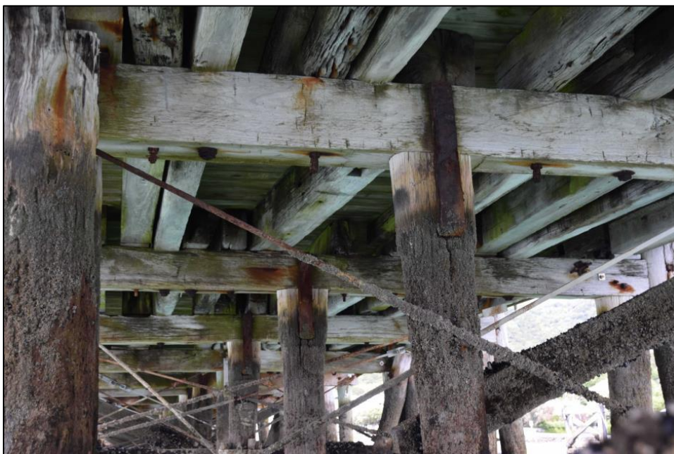
Figure 82. Original wrought iron strap connections between the central piles and their pile cap. The joints also have a mortise and tenon (Origin 2021).
