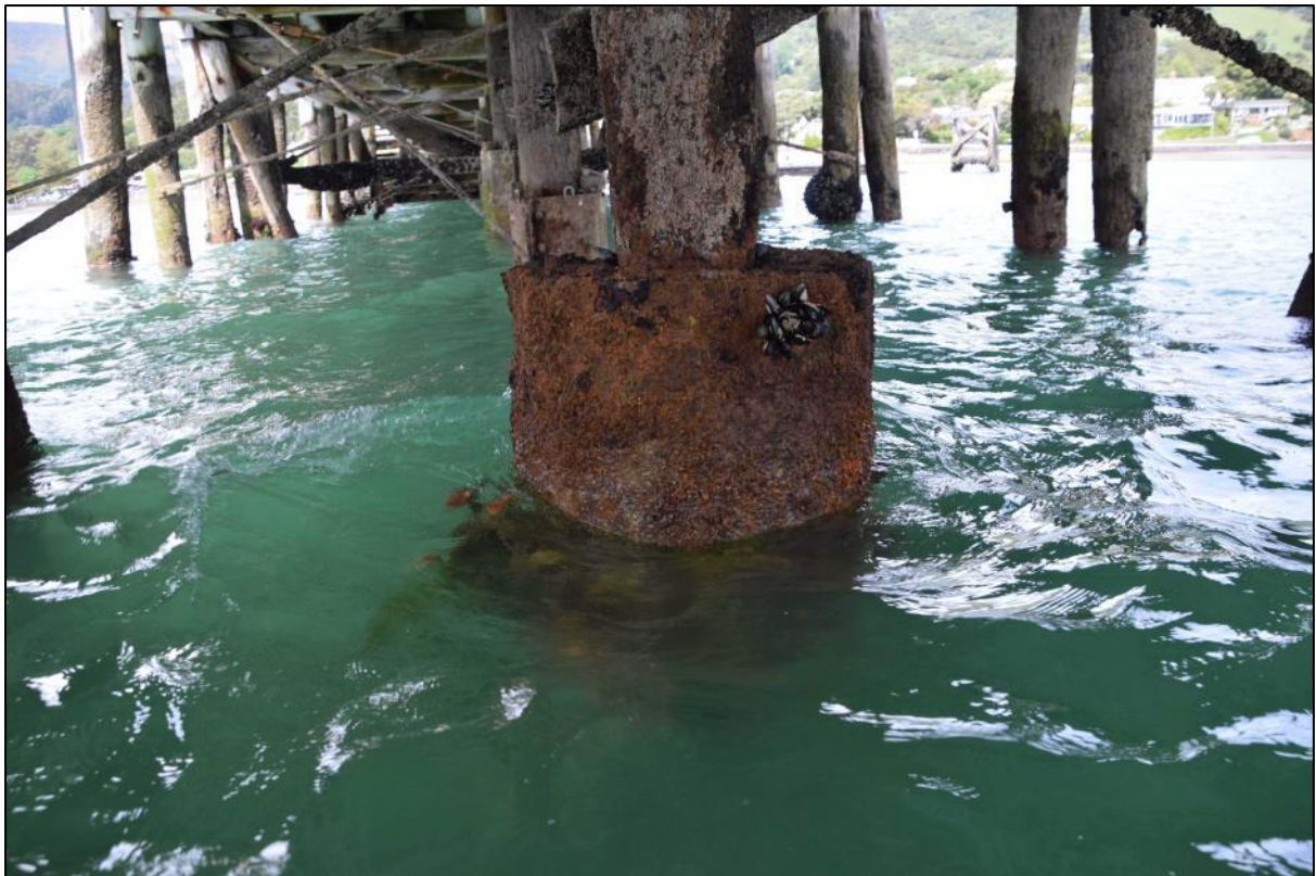
Photo 26 A 'jacket' repair to a central pile under the western end of the wharf. The pile has continued to erode above the jacket.
