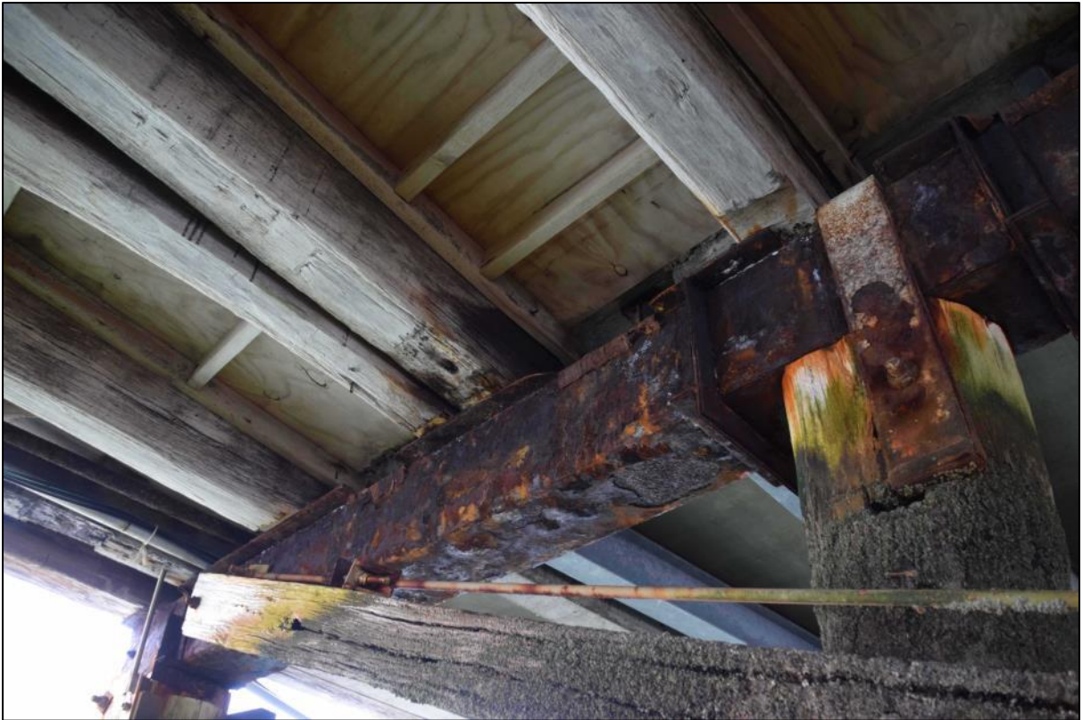
Photo 38 Severe corrosion to a past steel repair.
