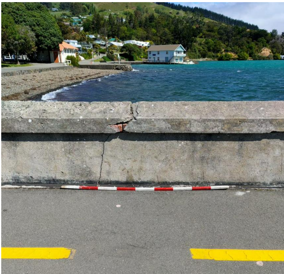
Figure 71. View of cracked portion of concrete parapet wall. Cracked portion of chamfered pier caps suggests it is composed of red brick with concrete render overlay. Image was taken looking south. Source: SIA 2021.
