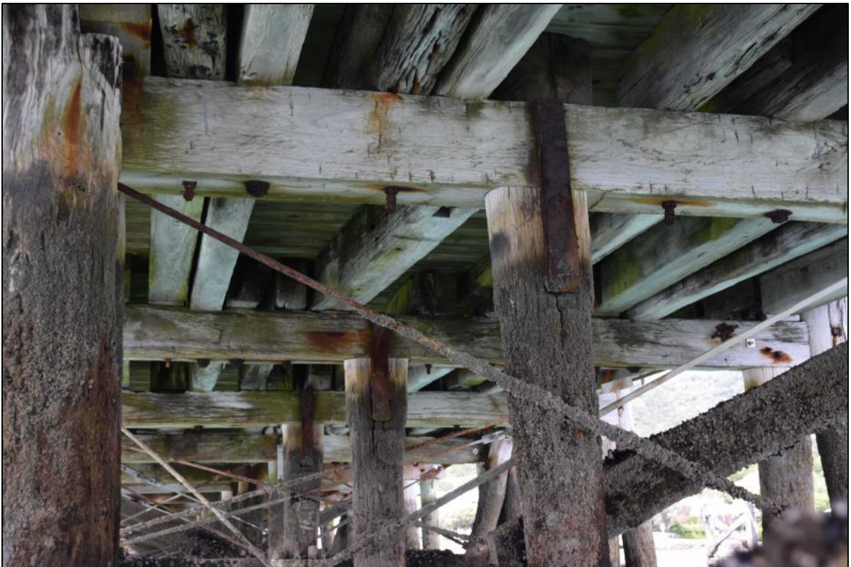
Photo 29 original wrought iron strap connections between the central piles and their pile cap. The joints also have a mortise and tenon.
