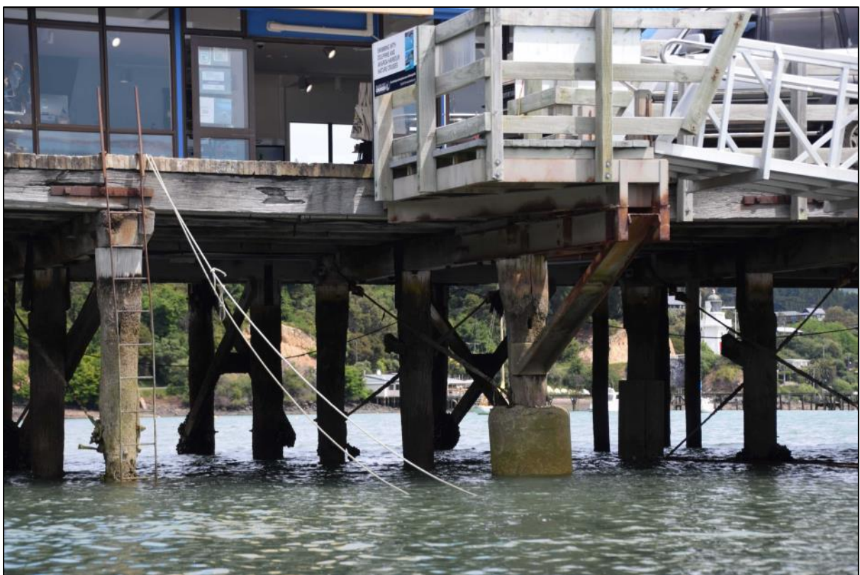
Photo 7 Further alterations on the north side of the wharf with steel added to support the gantry to the floating pontoon and concrete cast to the base of the pile supporting the steel framing.
