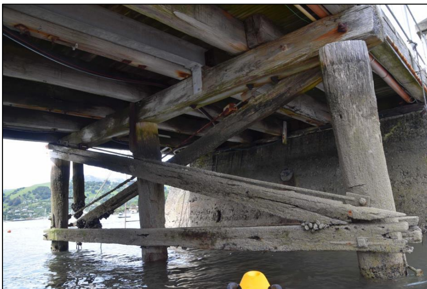
Figure 75. The first bent and the stringer/deck connection to the abutment. This part of the structure contains many original elements, including the pile cap, central pile with wrought iron strap connection to the cap, bracing timbers and horizontal wale between the piles, and timber stringers between the pile cap and modern decking boards (Origin 2021).
