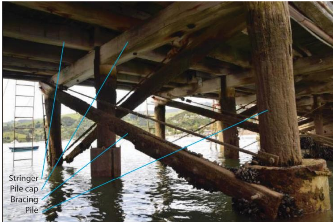
Figure 7. Another example of a 'bent' – the entire frame comprising, this time, three piles with a capping beam on top and bracing to provide rigidity. Source: Origin 2021.
