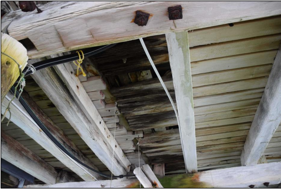
Figure 83. Decay in decking boards beneath the existing deck finish. Corrosion to original iron bolts and nuts (Origin 2021).
