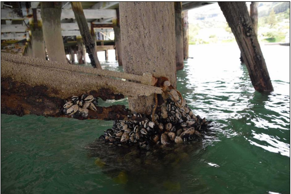
Photo 35 Broken/corroded steel brace.
