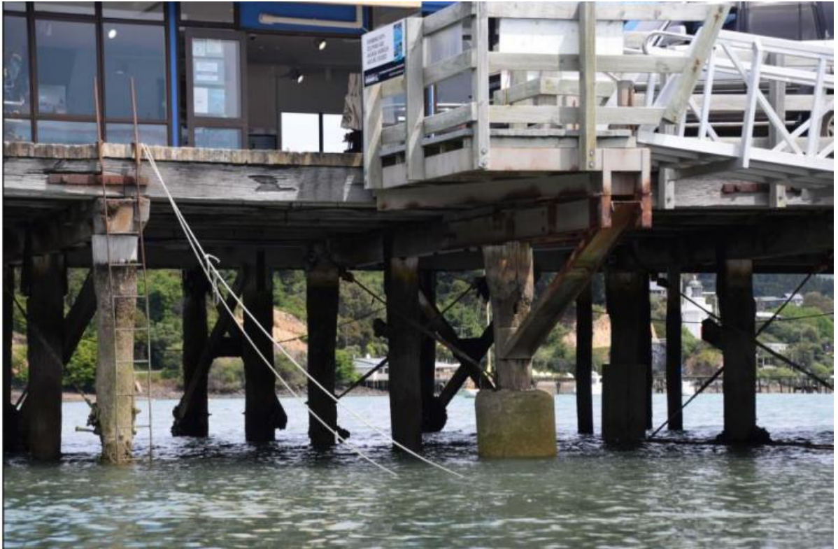
Figure 86. Alterations on the north side of the wharf with steel added to support the gantry to the floating pontoon and concrete cast to the base of the pile supporting the steel framing (Origin 2021).
