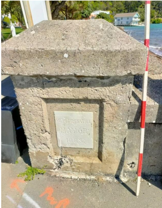
Figure 70. View of marble date plaque with the name of the Mayor, W. B. Tosswill. The incised letters and small drill holes indicate that the plaque should have lead lettering, and this has either fallen out or been removed. The image was taken looking south. Source: SIA 2021.
