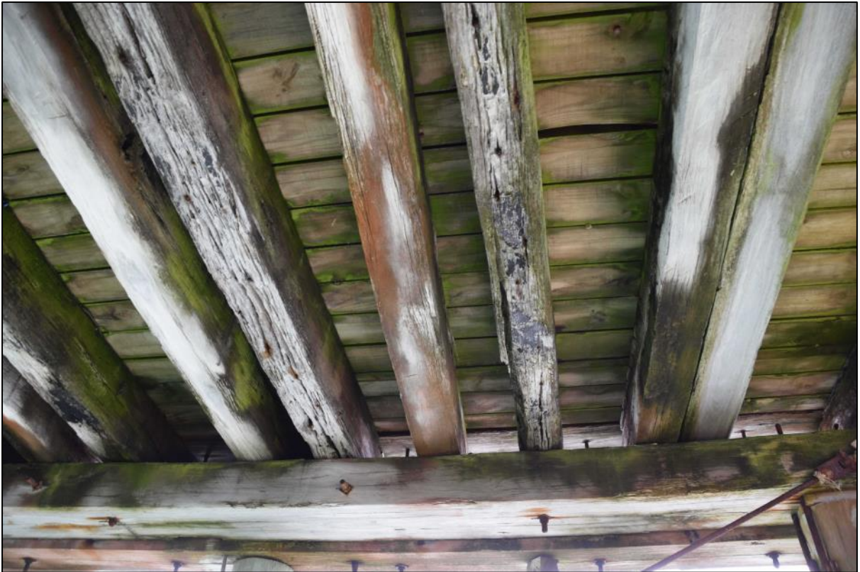
Photo 28 Additional stringers inserted to strengthen the deck at the western end of the wharf. There is considerable erosion and decay in many of the stringers here.
