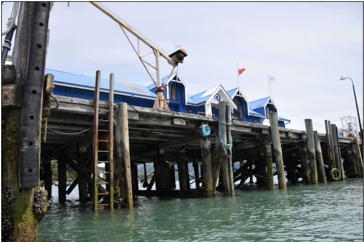
Photo 8 The north side of the wharf beyond the floating pontoon with modern ladders and replacement tanalised fender piles. The width of the wharf has substantially widened to accommodate the late 20th century sheds. Refer to Photo 9 below regarding the pile in the foreground on the left of the image.
