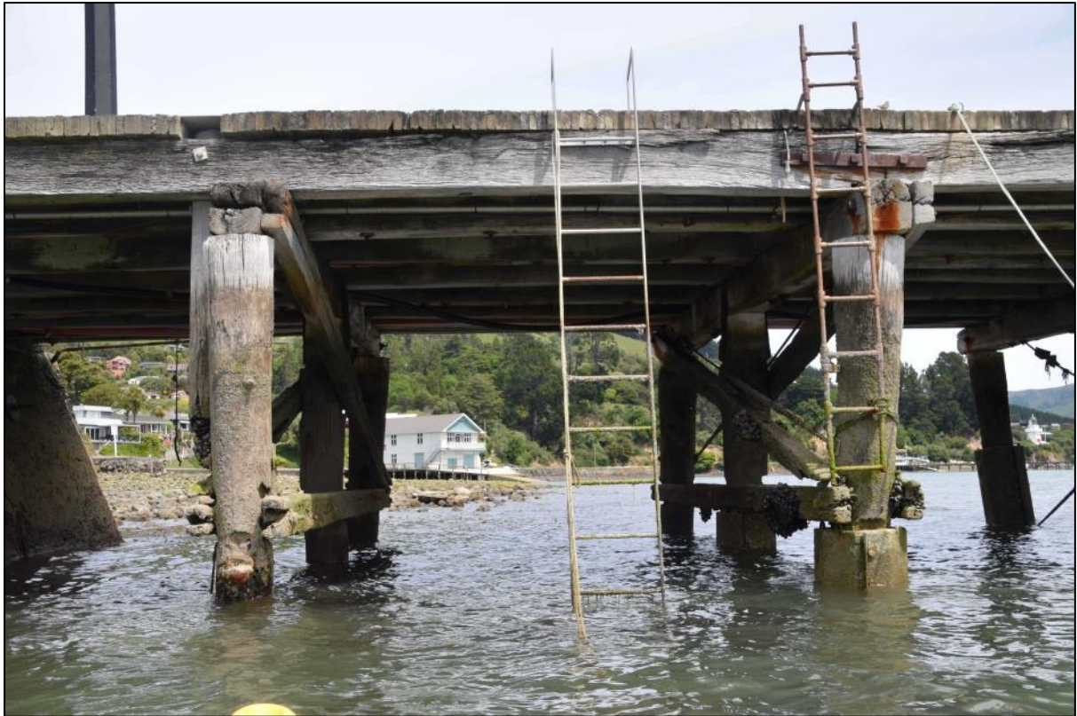
Figure 76. Three pile 'bents' under the eastern end of the wharf close to the abutment. Note the diagonal, timber braces, horizontal timber ties beneath the braces, and later steel rod braces. The original construction can be clearly seen here with timber pile caps (beams) running along the heads of the three piles in each bent and the timber stringers and decking on top. There are no fender piles to this part of the wharf. Ladders are a late 20th century addition (Origin 2021).
