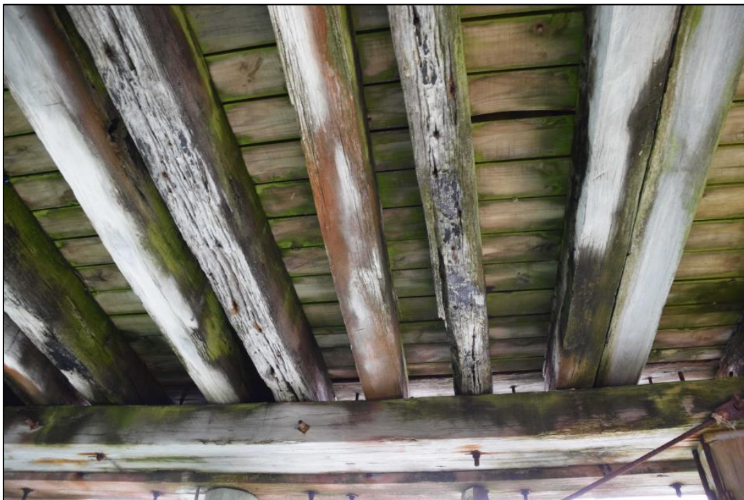
Figure 78. Additional stringers inserted to strengthen the deck at the western end of the wharf. There is considerable erosion and decay in many of the stringers here (Origin 2021).
