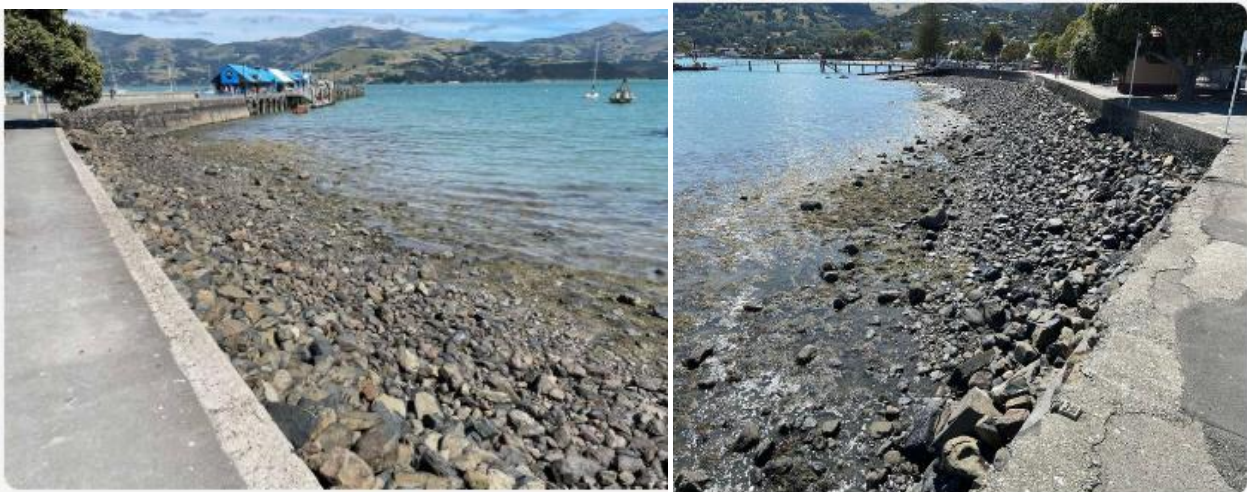
Figure 3.1: Placed and natural rocks along seawalls on the north side of the Akaroa main wharf.
