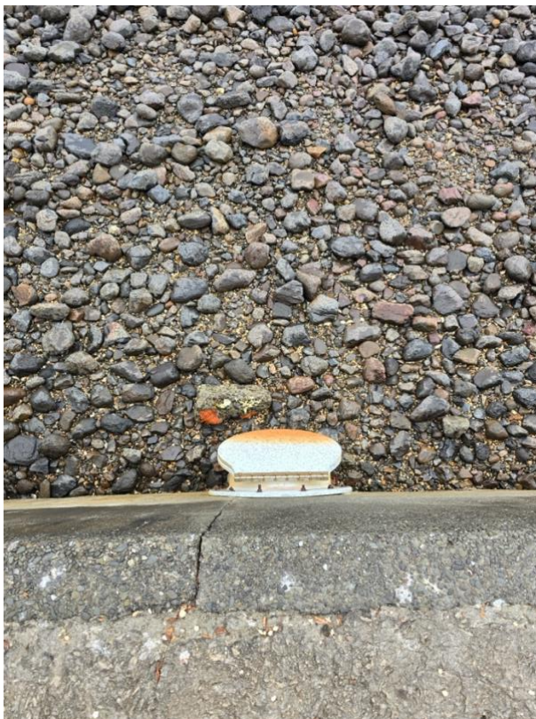
Figure 11 Examples of existing stormwater discharge and erosion protection at discharge points
