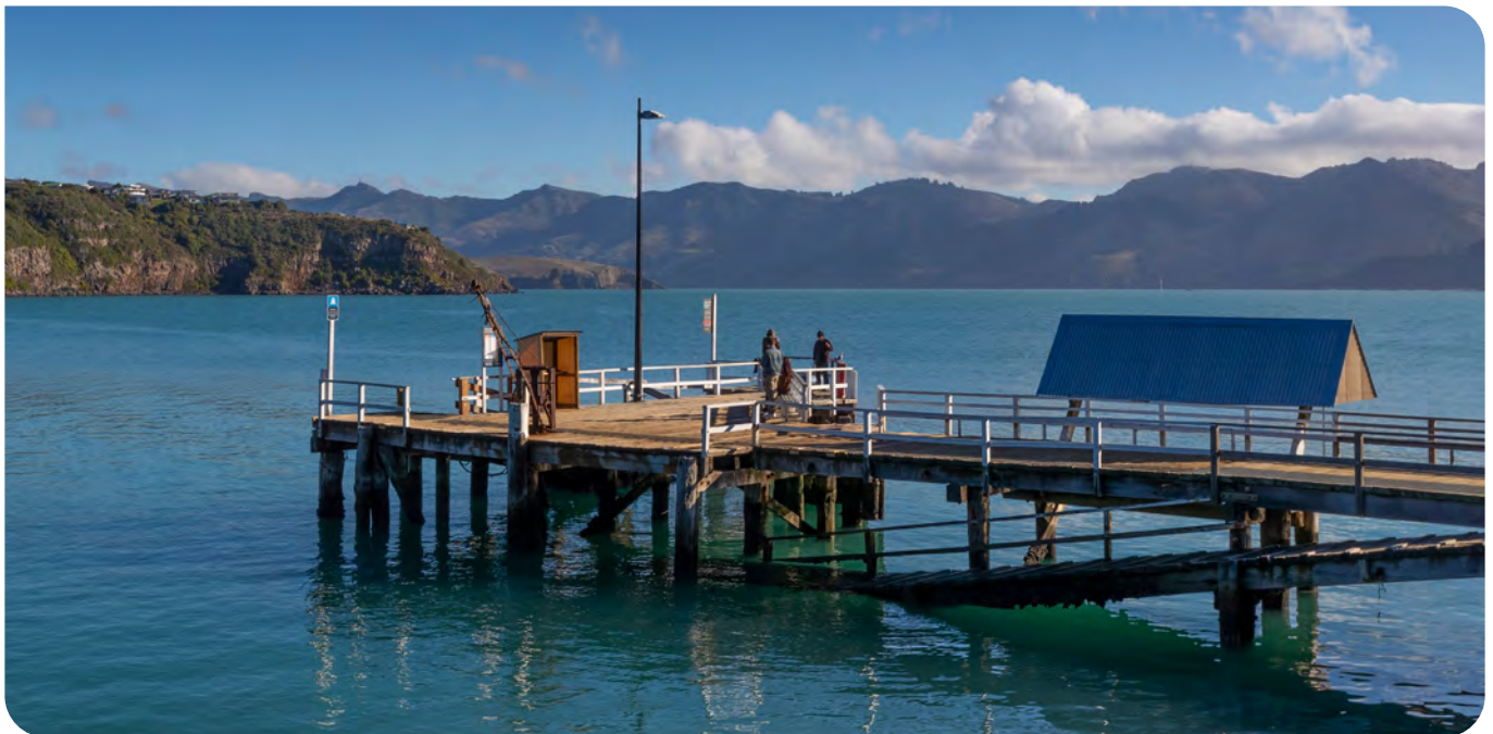
Diamond Harbour Wharf
