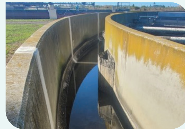
Clarifier - after repairs
