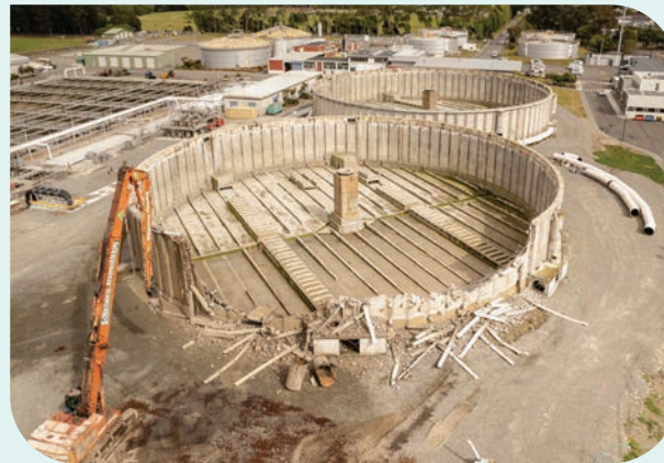
Demolition of the trickling filter tanks.
